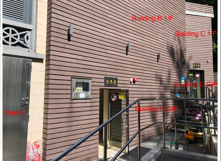
Photo 2: Building B and Wall A.
