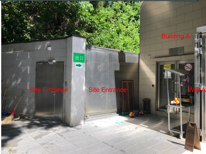
Photo 1: Entrance of the site and Building A.
