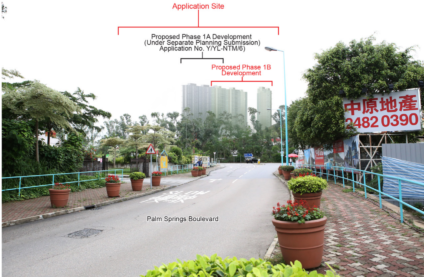
Proposed Scheme – Interim Scenario (Phase 1B Development and Phase 1A Development (Under Separate Planning Submission) (Application No. Y/YL-NTM/6))
