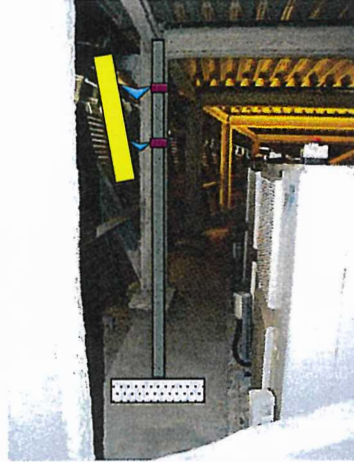
A2 antenna mounting detail
