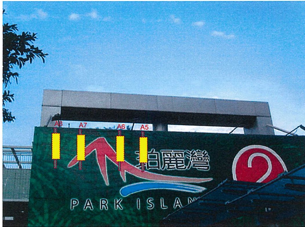
A5 ~ A8 Antennae will be mounted on the existing stainless steel frame behind the back-drop Location
