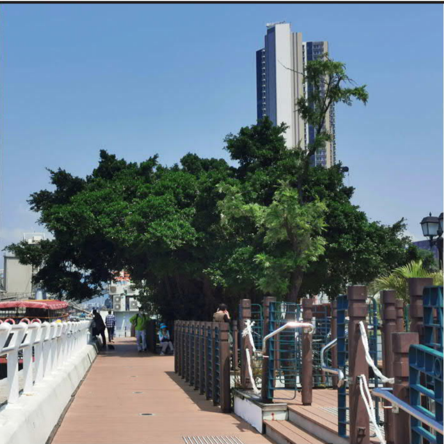
Photo H1 Existing Conditions of the Subject Site (Before)
