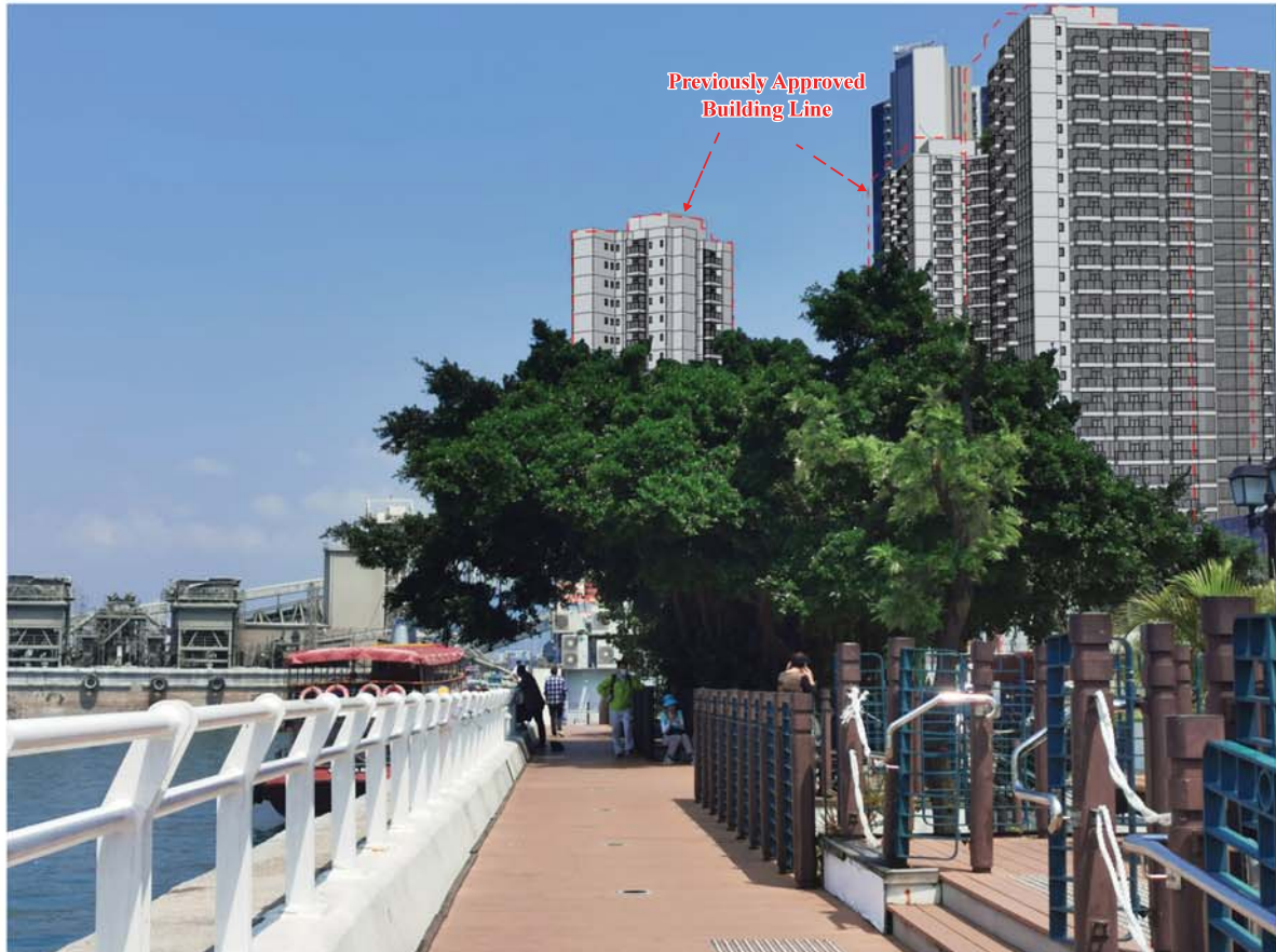
Photo H2 Proposed Development at the Subject Site
