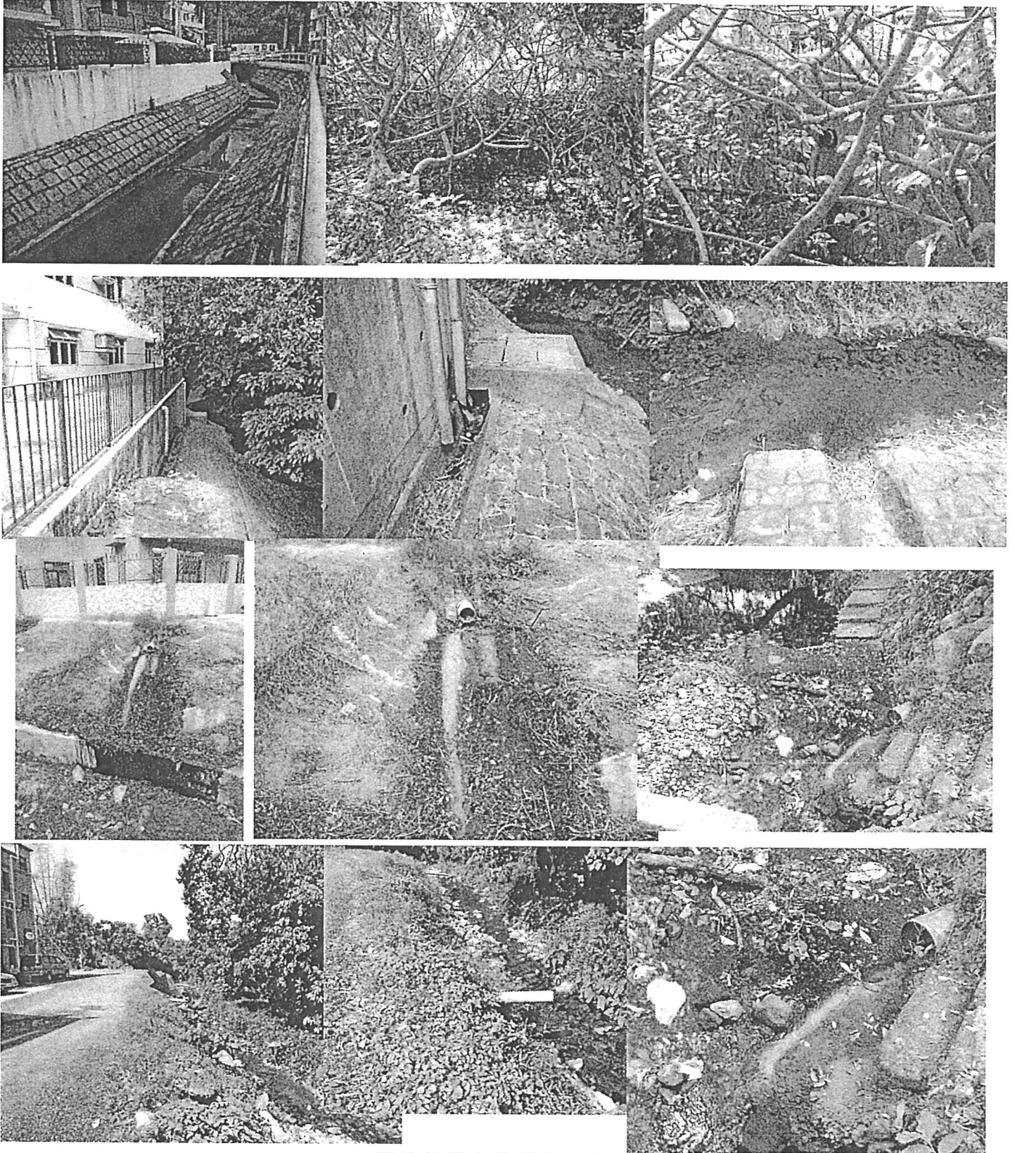
Figure 3. Pipes discharging wastewater/ grey water along watercourses next to village areas
