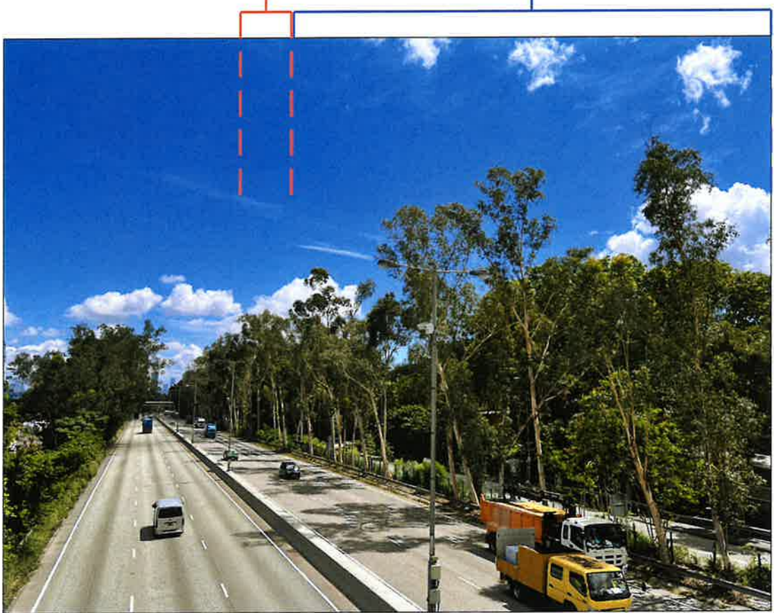
Existing condition (Scheme A)
