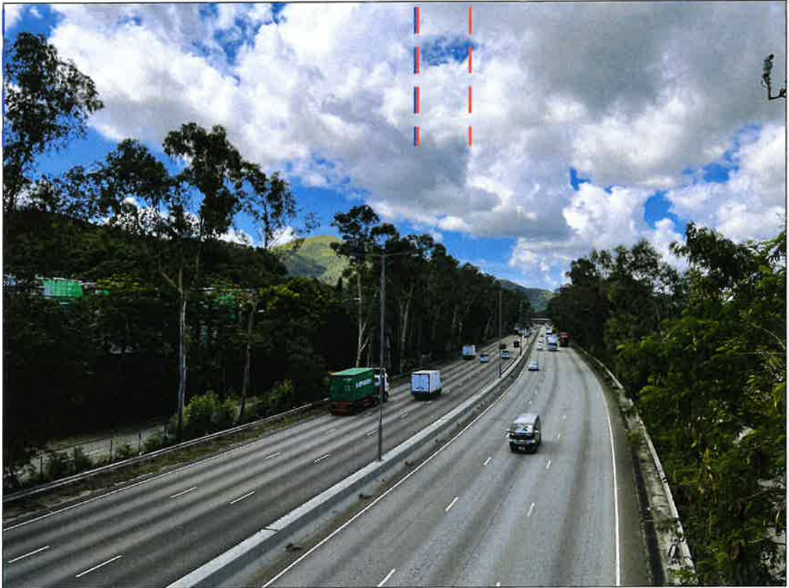
Existing condition (Scheme A)
