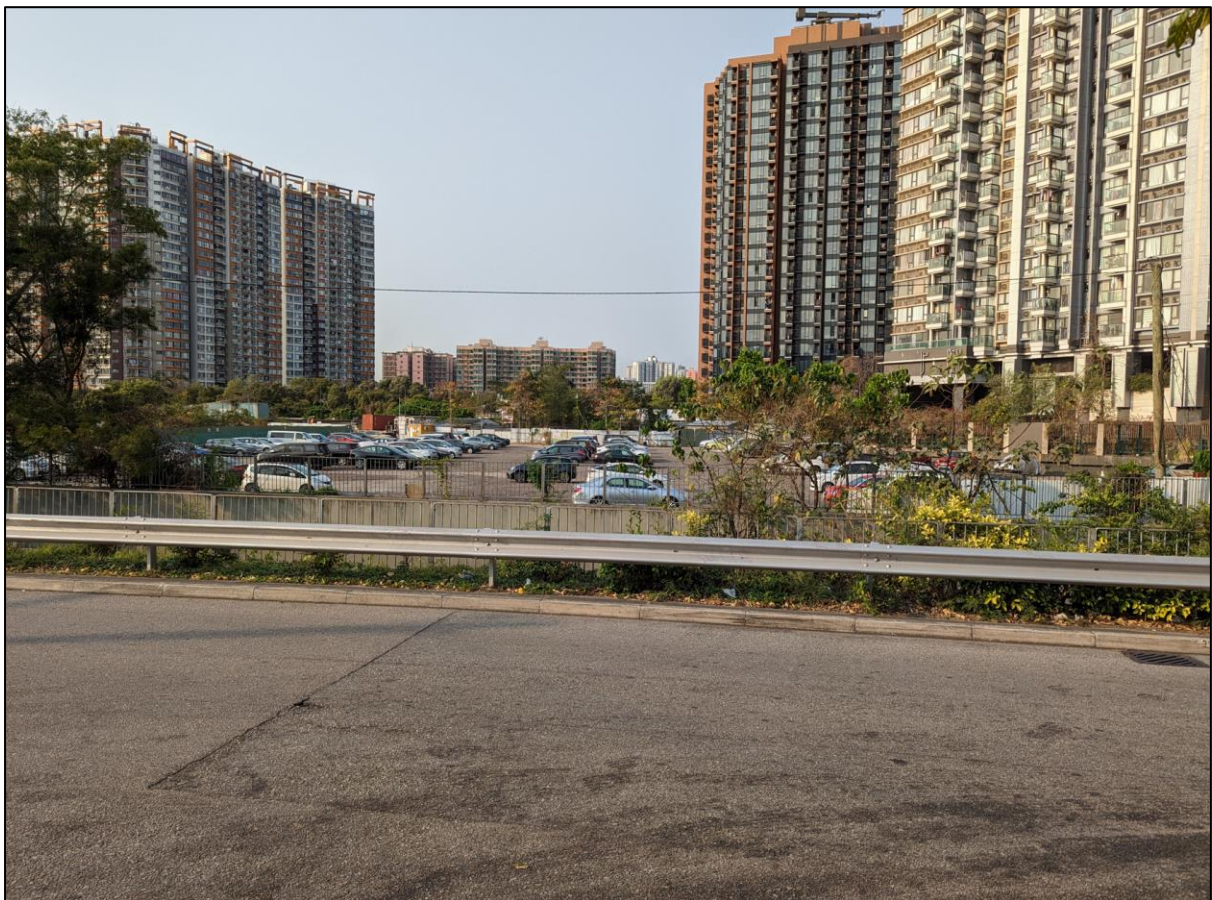
NS 06b Open Parking at the Southwest of the Site (From Lam Hi Road)
