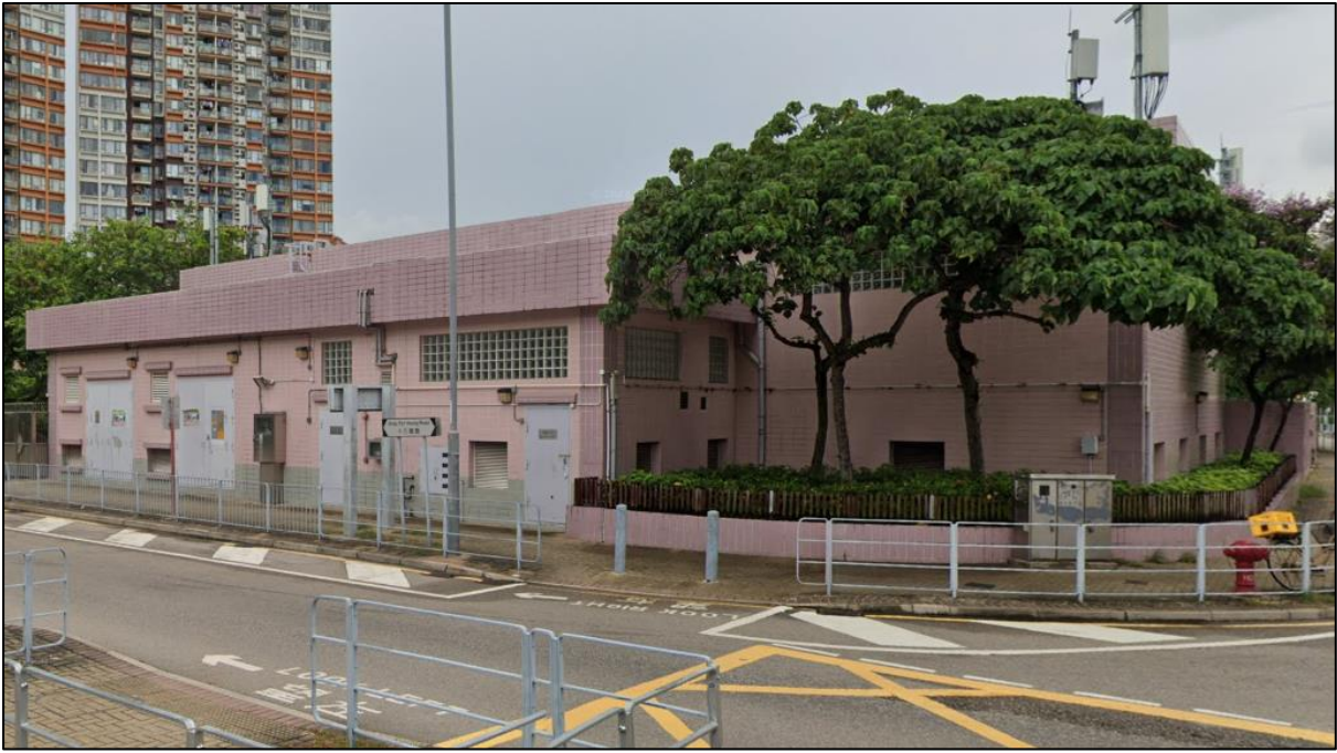
NS 01: Ma Tin Sewage Pumping Station
