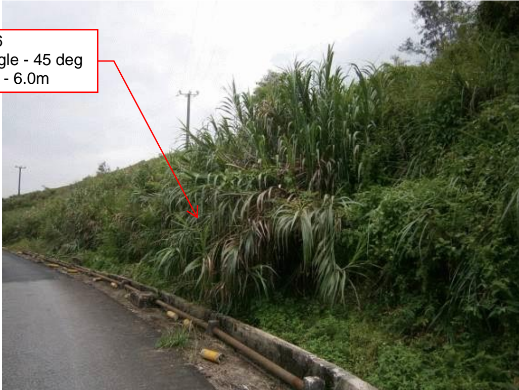
Photo 1: General View of 2SE-B/C296
