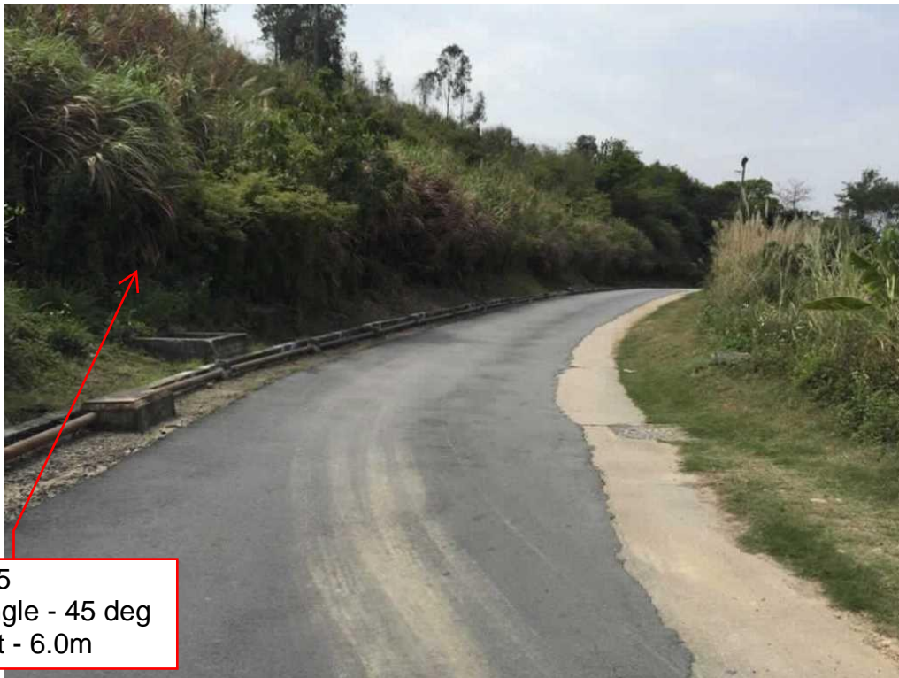
Photo 2: General View of 2SE-B/C305
