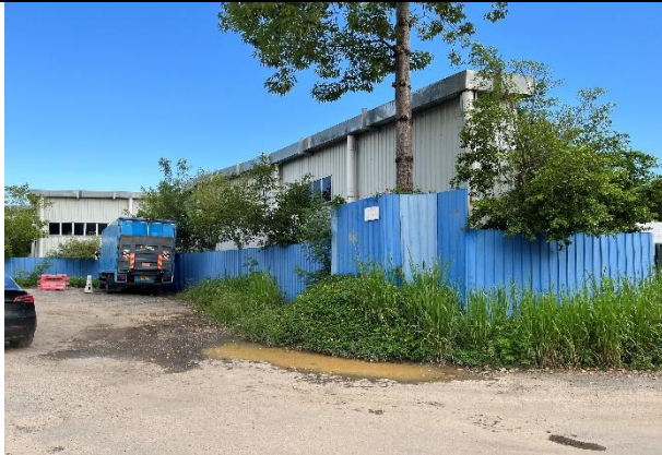
Photo 11: Building structure of warehouse to the North East of the Project Site
