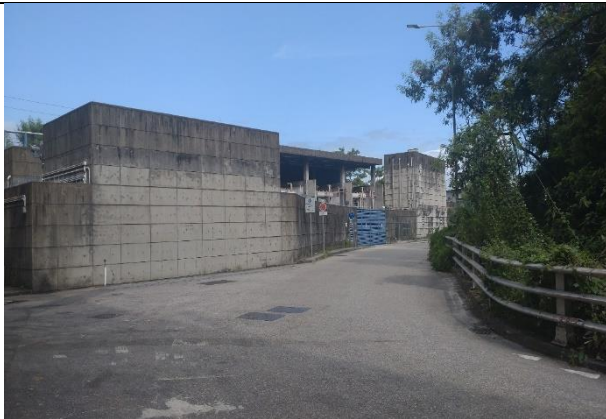
Photo 7: Tin Shui Wai West Rail Substation
