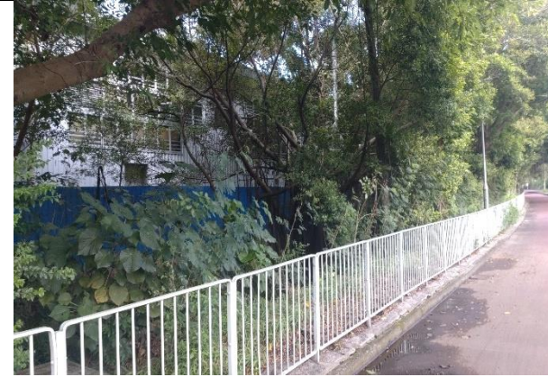
Photo 10: Building structure of warehouse to the North East of the Project Site
