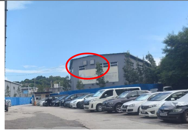
Photo 2: Louvers at Warehouse (VANPAC Group Asia)
