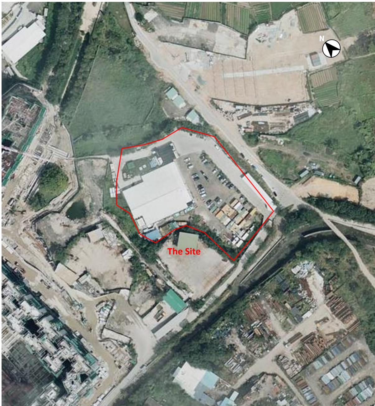
Figure D-6 Aerial Photograph in Year 2015
