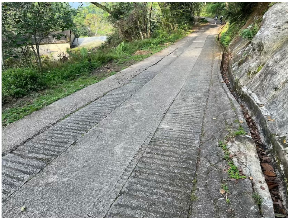
Plate 6 – Access Road and 300mm U-channel
