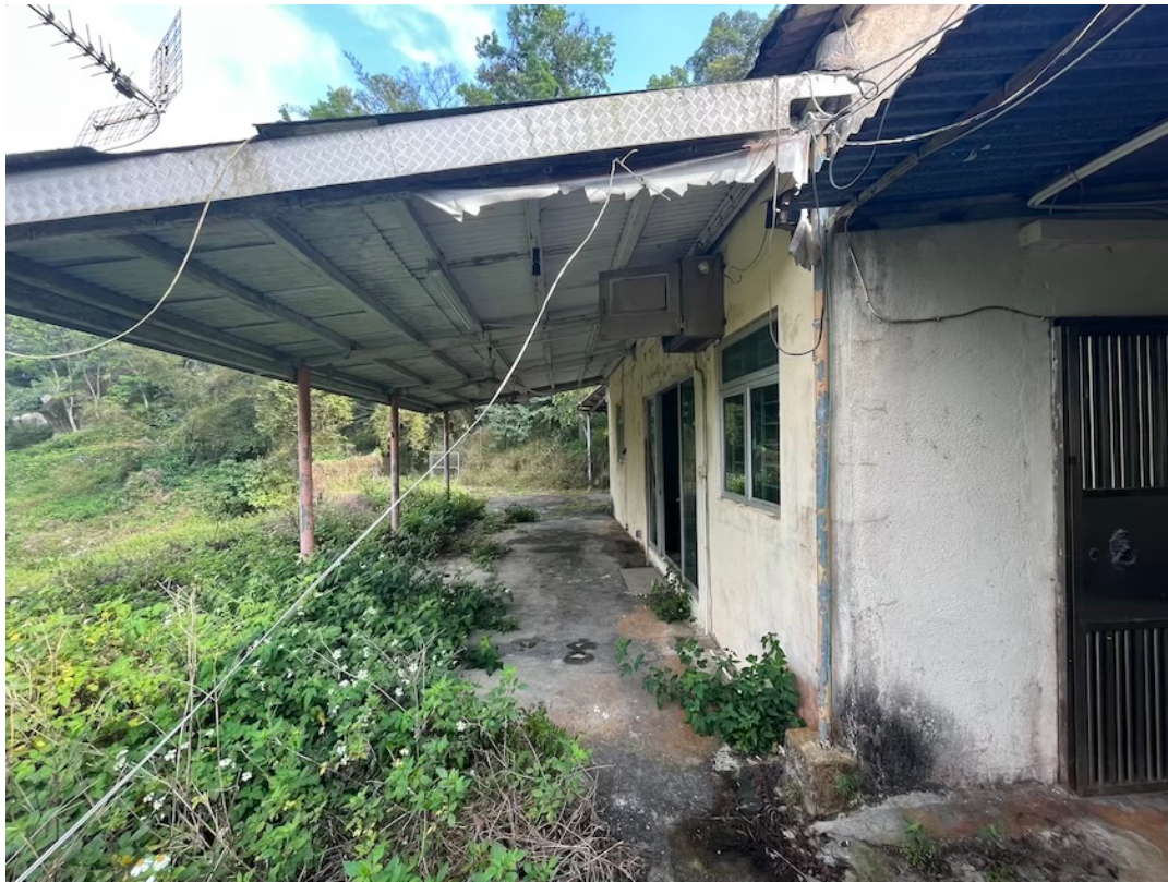
Plate 3 – Existing Building and Paving
