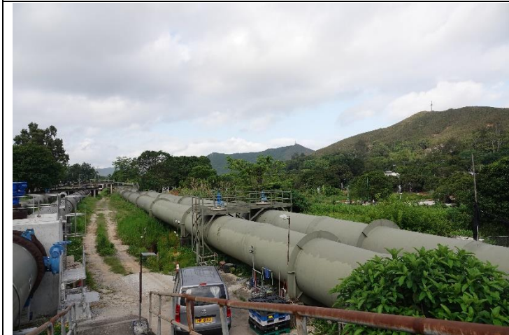
Photo 3. General View of Subject Site
