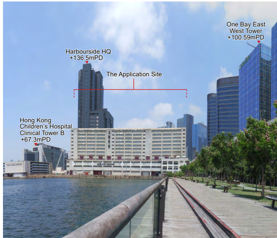
Existing View View northwest from Kwun Tong Promenade towards the Site
