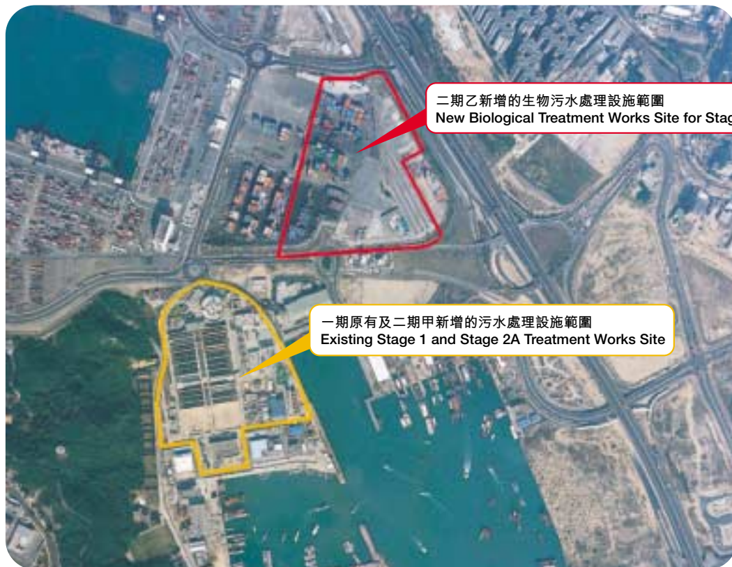
▲ 昂船洲污水處理廠位置 The Stonecutters Island Sewage Treatment Works Site
