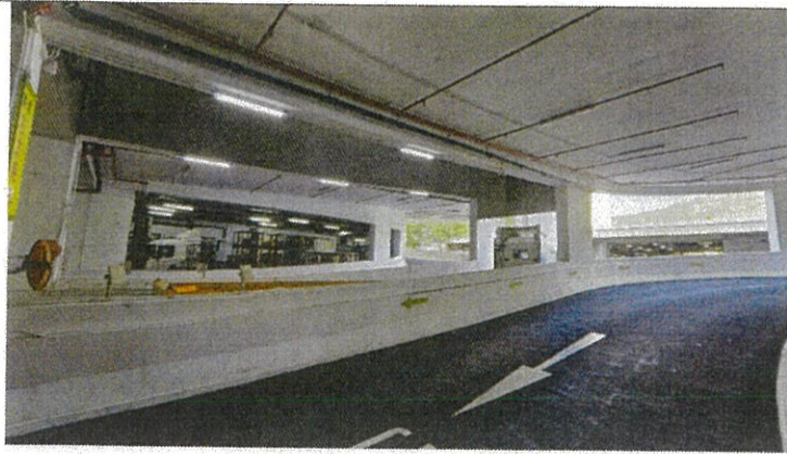
Fig 4a. CO 2 refilling area next to car ramp on G/F
