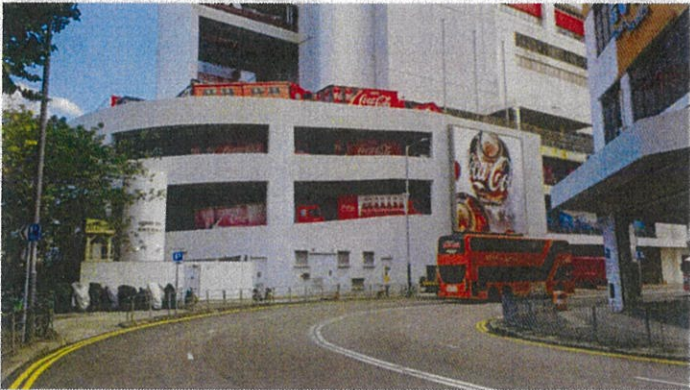
Fig 2. Semi Open-air car ramp for delivery trucks and vehicles from G/F to 3/F
