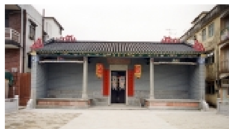
King Law Ka Shuk, Tai Po after restoration
