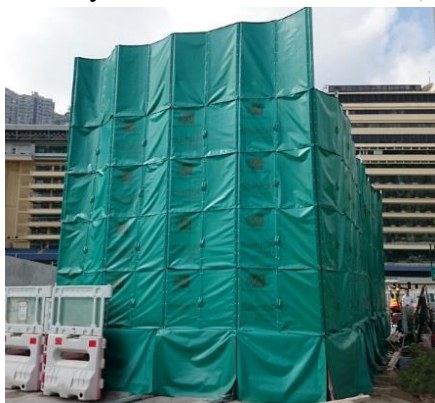
Figure 5.15 Noise barrier (modular reusable, courtesy of Acoustics Innovation)
