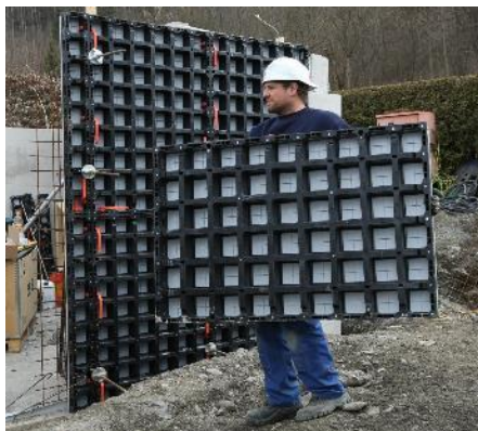
Modular Lightweight Formwork
