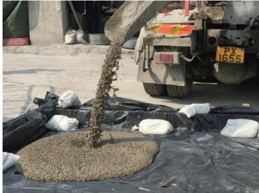
Self-compacting Concrete (Courtesy of Gammon Construction)
