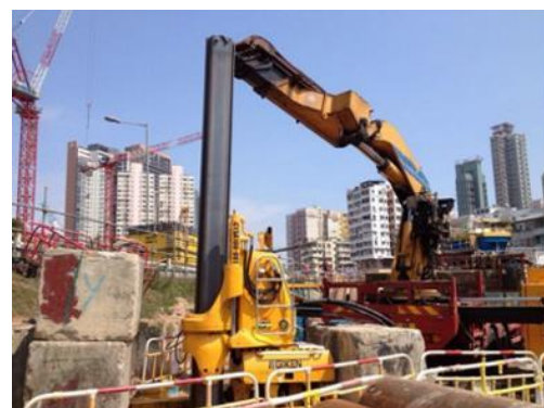
Press-in Piling Machine
