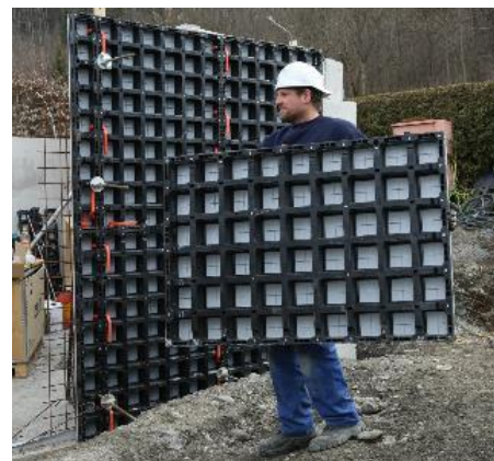
Modular Lightweight Formwork
