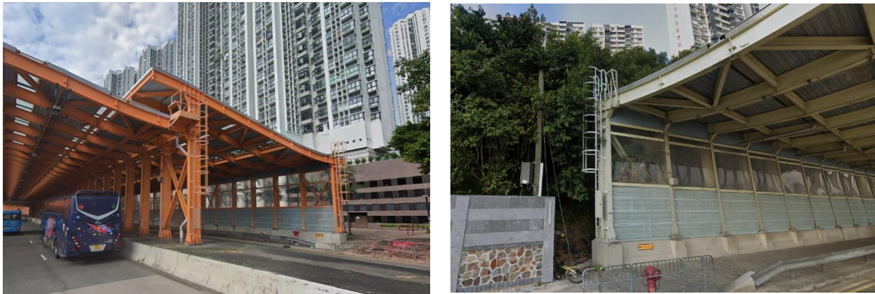
Figure 4.5.2 Access ladders on noise enclosure
