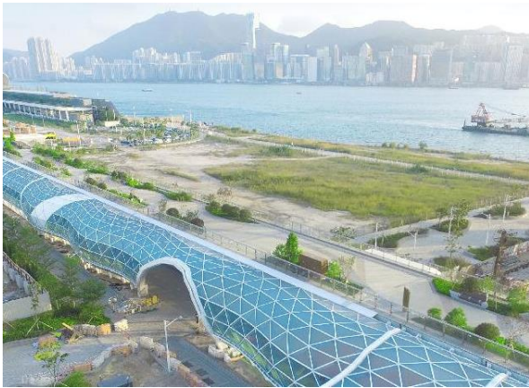
Noise enclosures with a curved and rippling design at Kai Tak, Hong Kong
