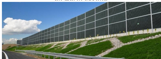
Figure 3.4.5 Example of Barrier Sitting on top of an Earth Mound
