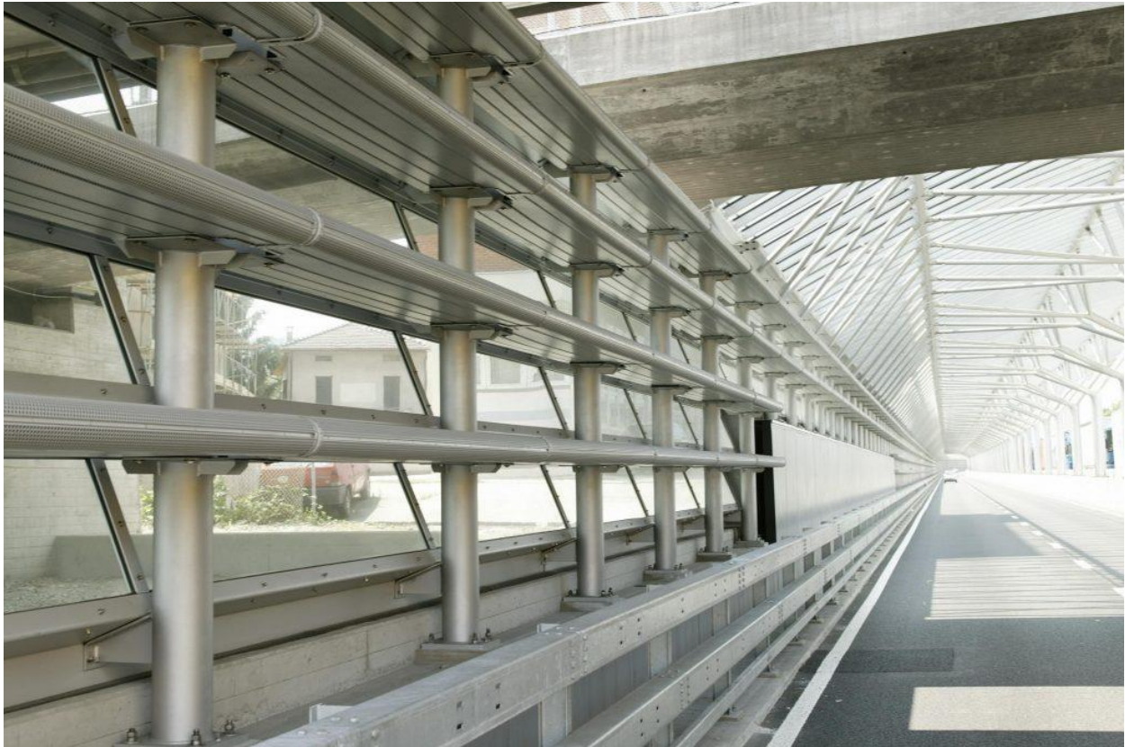
Figure 3.2.8(c) Example of Angled Noise Barrier Panel
