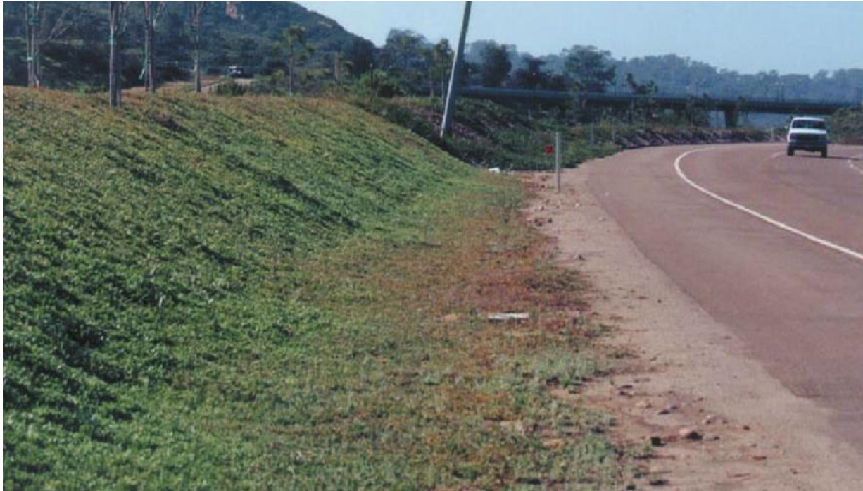
Figure 2.7.2 Example of Earth Berms
