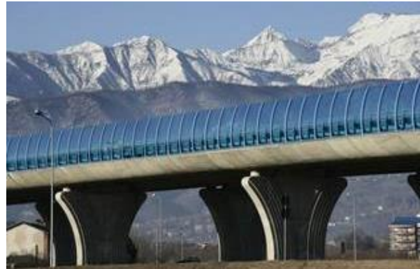
Colours used to accentuate the bridge
