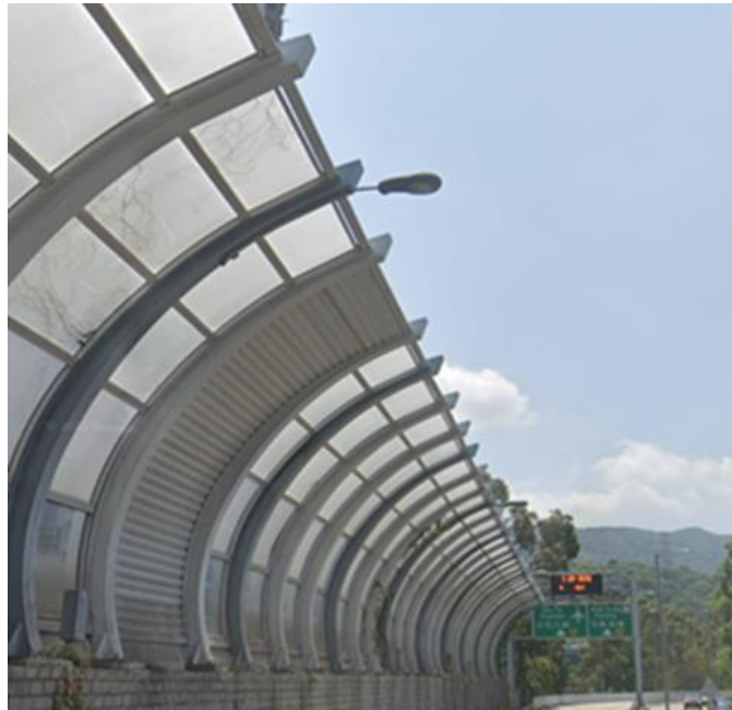
Lighting attached to noise barrier
