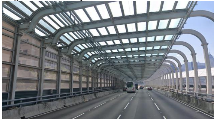
Figure 3.4.4 Transparent Panel in Semi-enclosure
