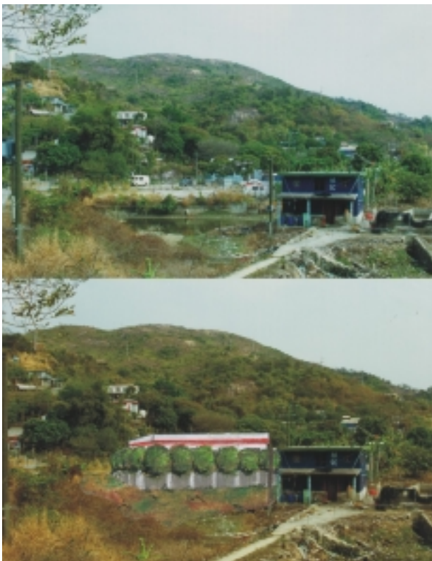
Photomontage of Tai Lam Valley Pumping Station – Before (upper) and at completion with mitigation (lower)
