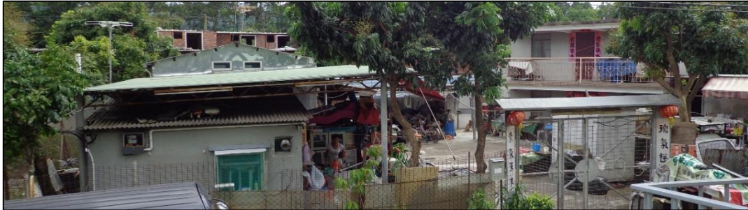
Existing village houses
