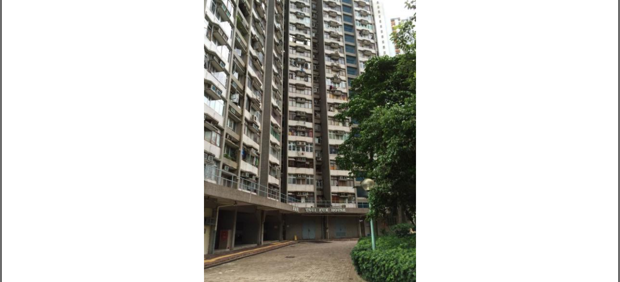
NSR 6 Tsui Fuk House, Tsui Wan Estate
