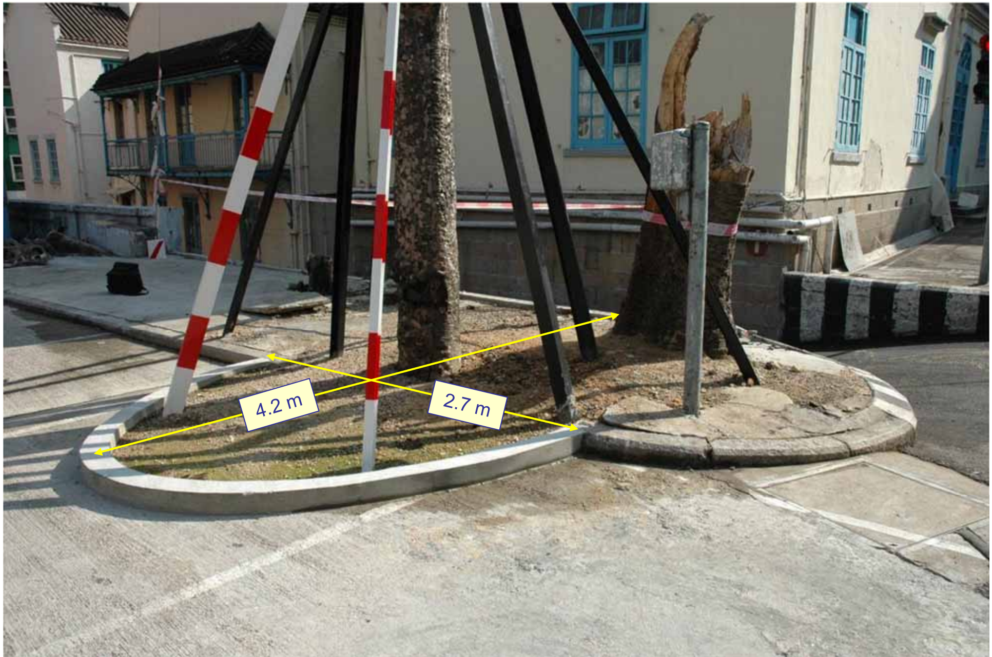
Figure 21. The original tiny tree pit of T3 has been enlarged in conjunction with the salvage operation conducted after Typhoon Fengshen.
