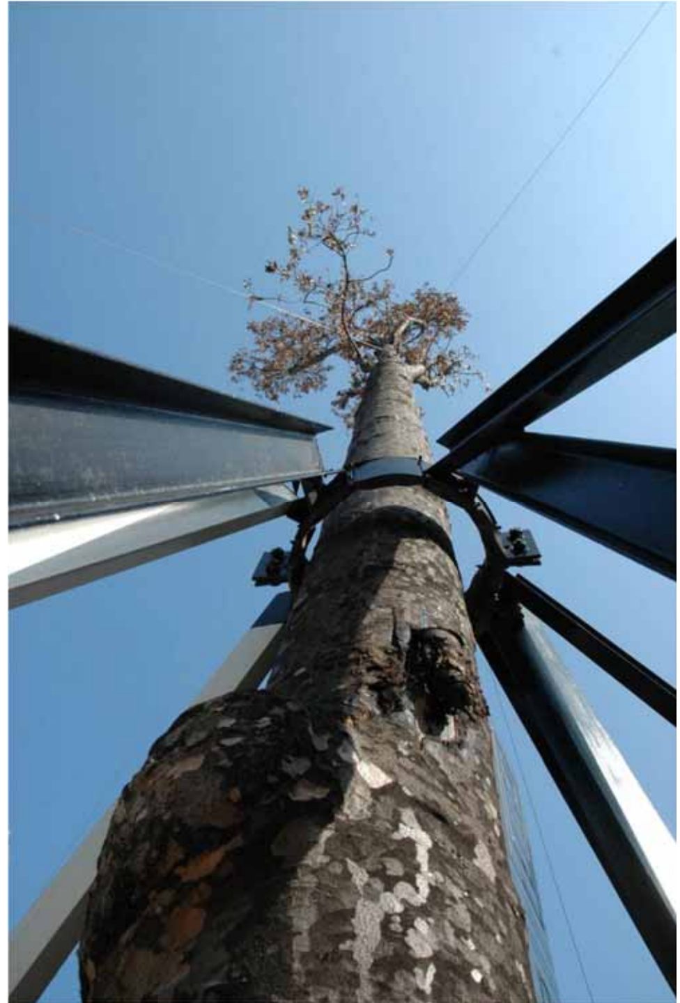
Figure 18. The tree prop supporting T3 has been designed to avoid physical contact with the trunk. Note the tiny amount of remnant branches and leaves, resulting in a crown ratio of merely about 10%.
