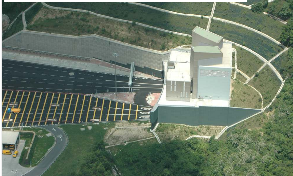
Completed Portal of Shatin Heights Tunnel
