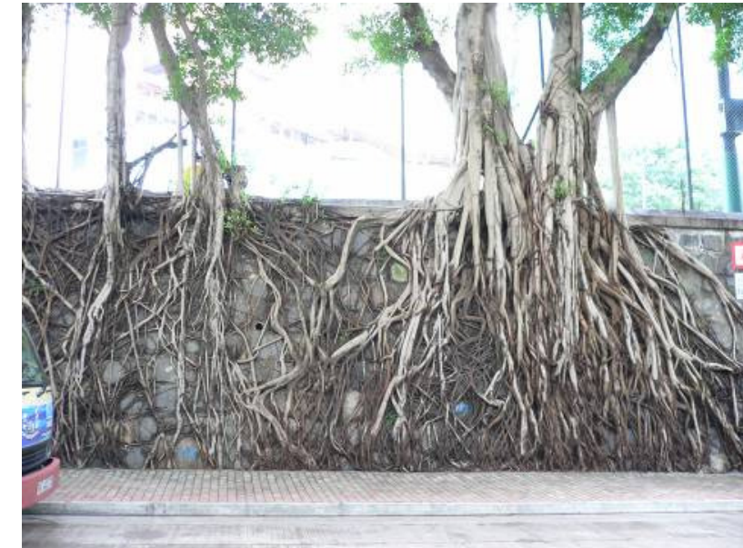
Fencing wall outside the Park (the main wall)
