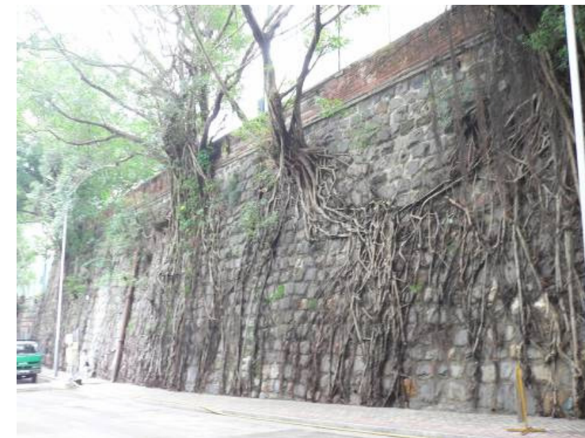
Masonry wall at the west perimeter of the playground
