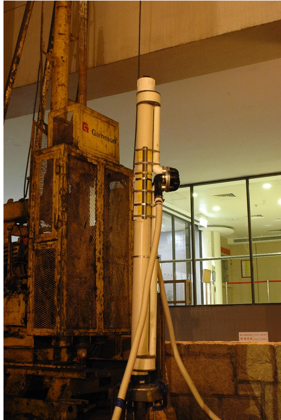
PHOTO 1 IMPACT HAMMER AND DOWNHOLE LOAD CELL ATTACHED, RESPECTIVELY, TO THE TOP AND BOTTOM OF THE DRILL STRING AT IMPACT BOREHOLE 024 INSIDE TSAN YUK HOSPITAL
