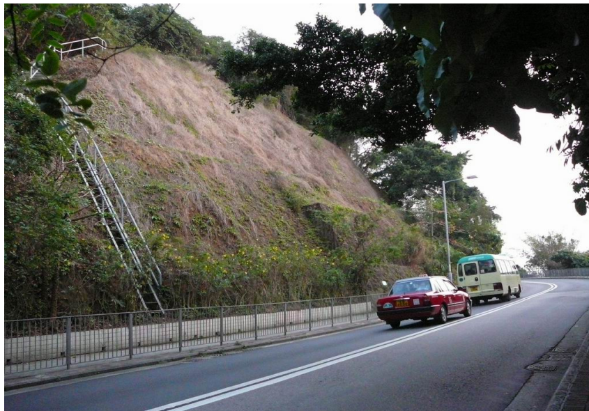
Developed Area (engineered slope along Victoria Road)
