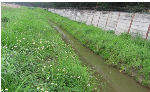
Plate 8.6 Drainage Channel/ Ditch
