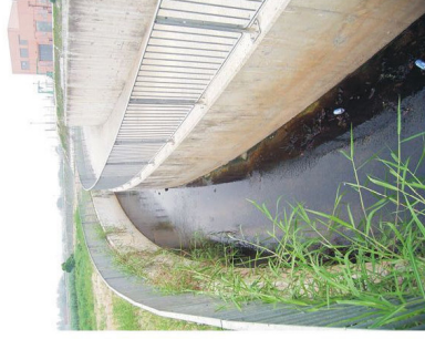
46. LR049 - Channel beside DSD building
