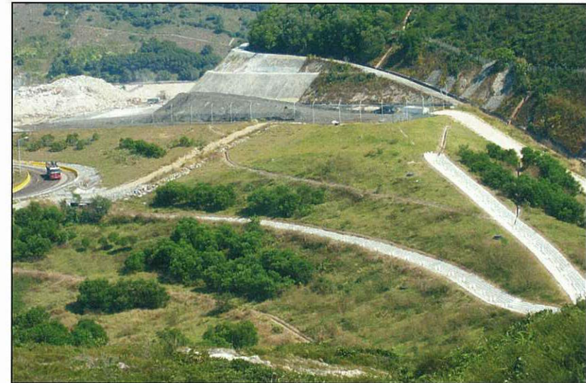
Some of the area within the existing SENT Landfill was hydroseeded as grassland.
