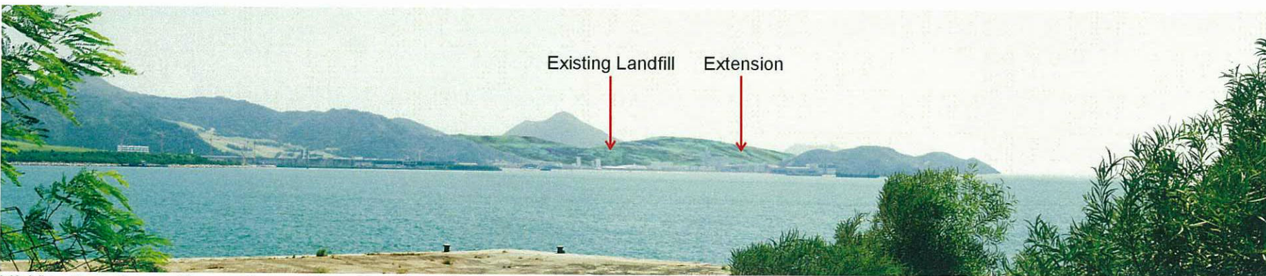
V3-View from Ocean Shores, Tseung Kwan O at Year 10 after full restoration
