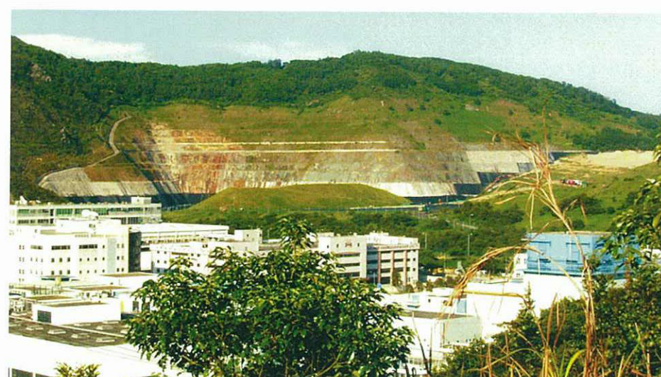
LR17 - Man-made slope with shrubs and grass in SENT Landfill
