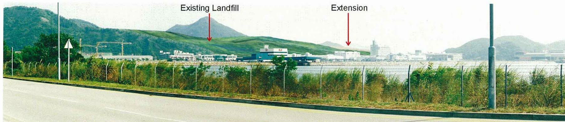
V8-View from Tseung Kwan O Area 86 at mid-point of operation
