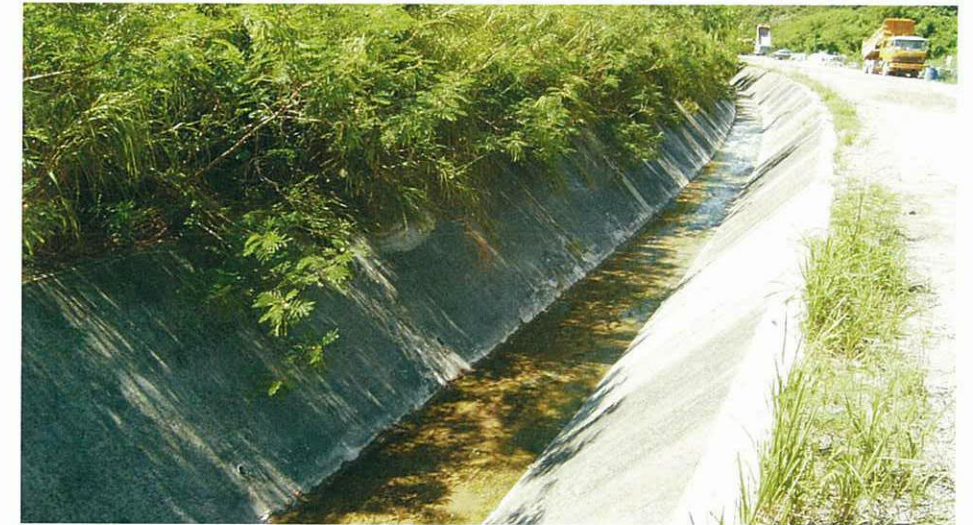
LR6 - Drainage channel in TKO Area 137
