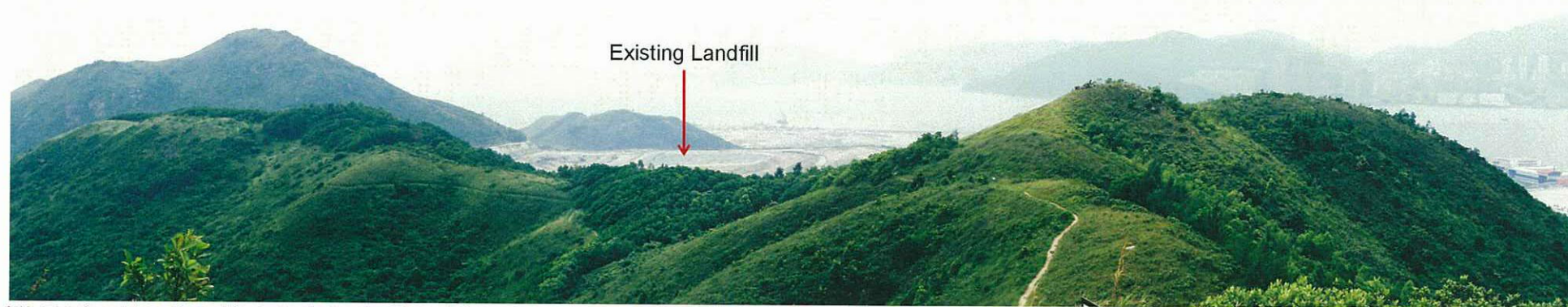
V4-Existing View from High Junk Peak, Clear Water Bay Peninsula
