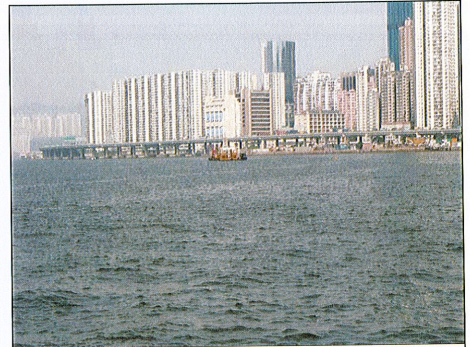
PHOTO C20 - T3 ISLAND EASTERN CORRIDOR
