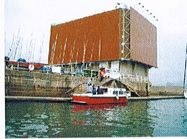
Vertical seawall nearby
