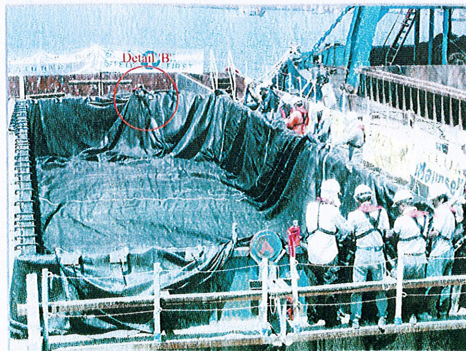
Two teams of worker sealing the container by hand stitching under the supervision of the site supervisors
