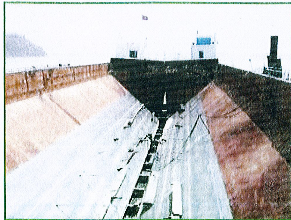
Split bottom hopper barge prior to installation of bulkheads
