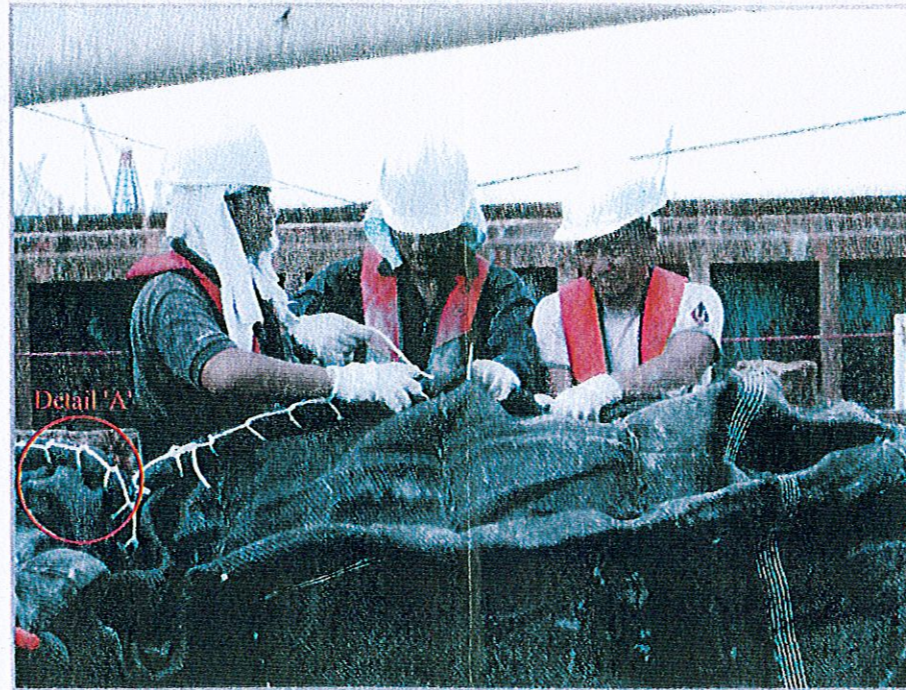
Sealing the container by hand stitching
