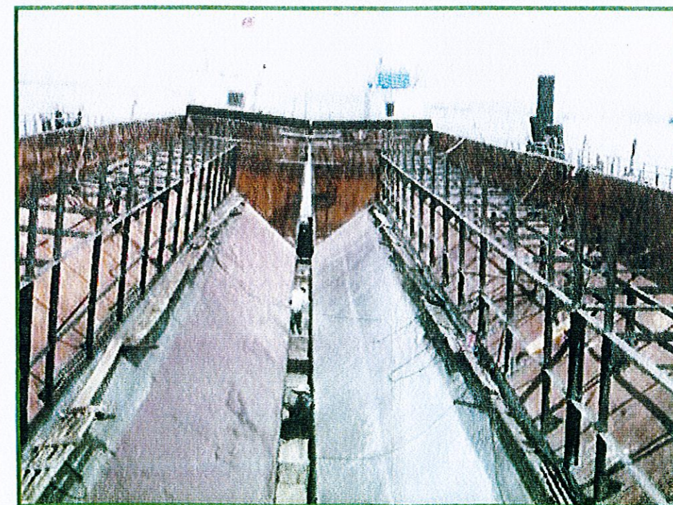
Installation of longitudinal bulkhead to the split bottom hopper barge
