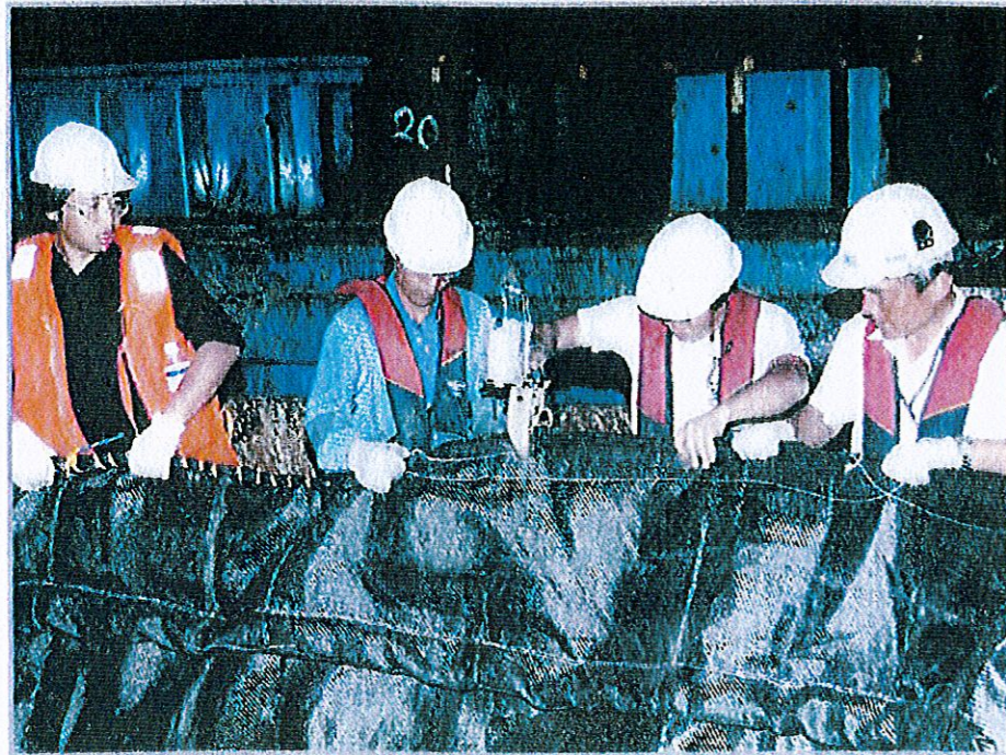
Sealing the container by sewing machine (Container A only)
