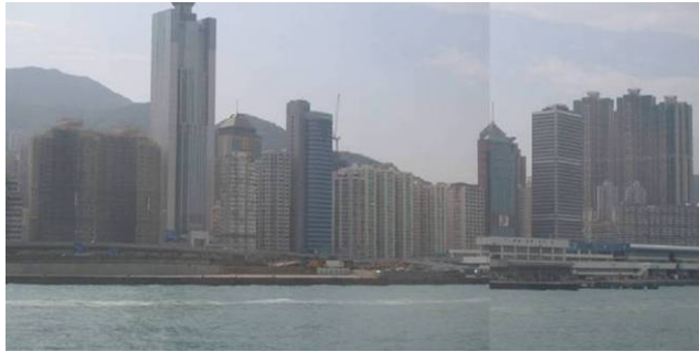
Wharf piles and vertical artificial seawall along the shore of Sai Ying Pun.
