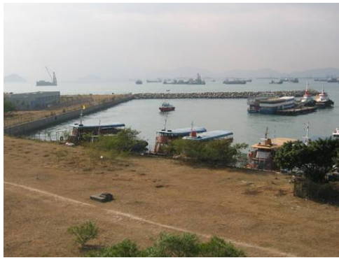
New Yau Ma Tei Typhoon Shelter with vertical artificial seawall and breakwaters at the coast.
