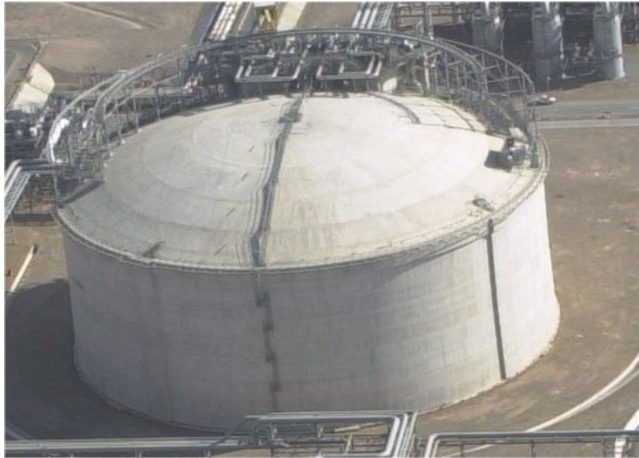
Figure 1.2 Typical LNG Storage Tank
