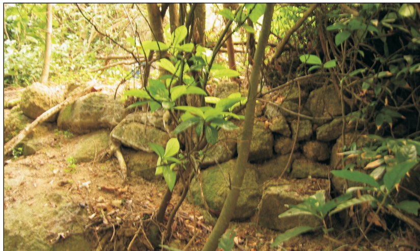
Granite Built Retaining Wall
