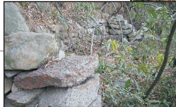
Stone Wall Structure of Structure 2b
