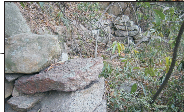
Stone Wall Structure of Structure 1b
