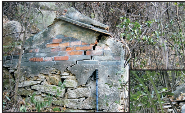
Gable of Building Structure 2a
