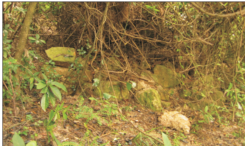
Granite Built Retaining Wall
