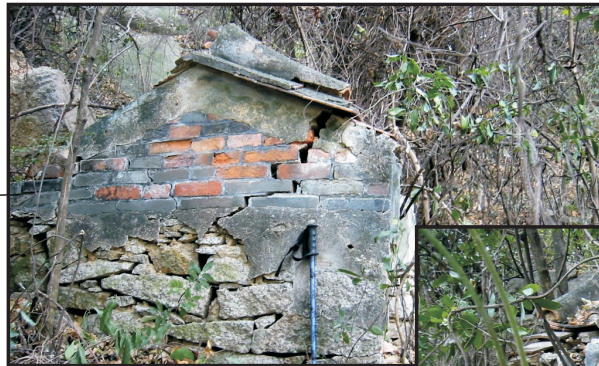
Gable of Building Structure 1a
