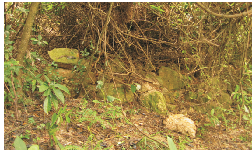
Granite Built Retaining Wall
