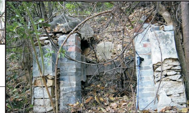
Facade of Building Structure 1a
