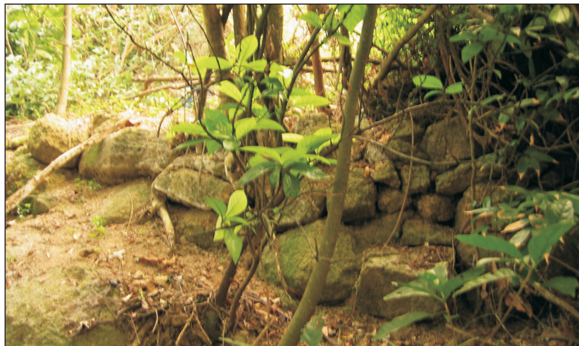
Granite Built Retaining Wall
