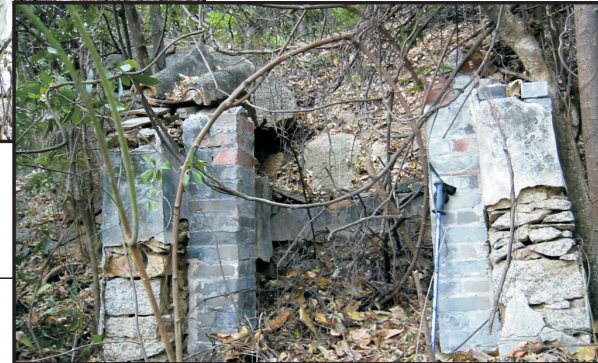
Facade of Building Structure 2a
