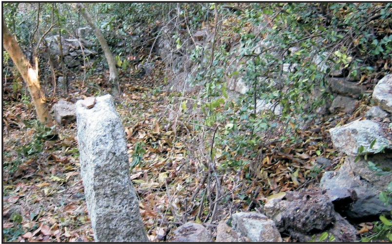
Stone Wall Structure
