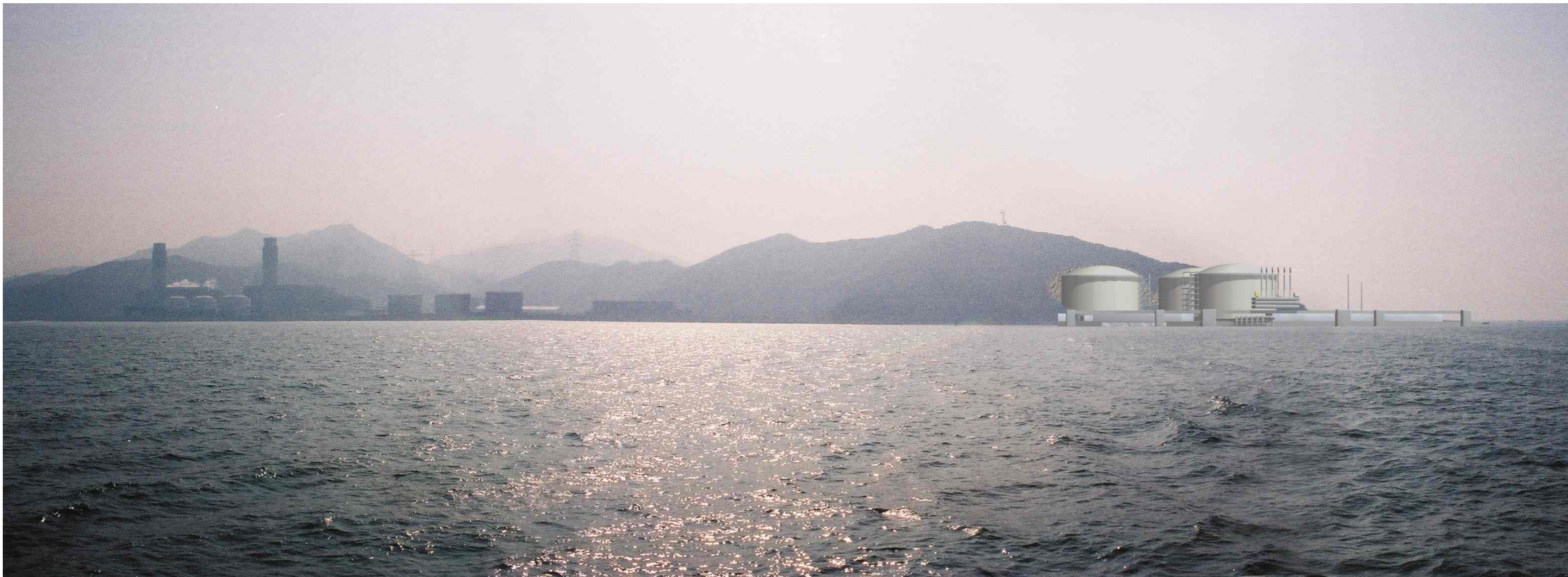
VIEW DISPLAYING THE 3D MODEL OF THE PROPOSED DEVELOPMENT YEAR 10 WITH MITIGATION MEASURES
