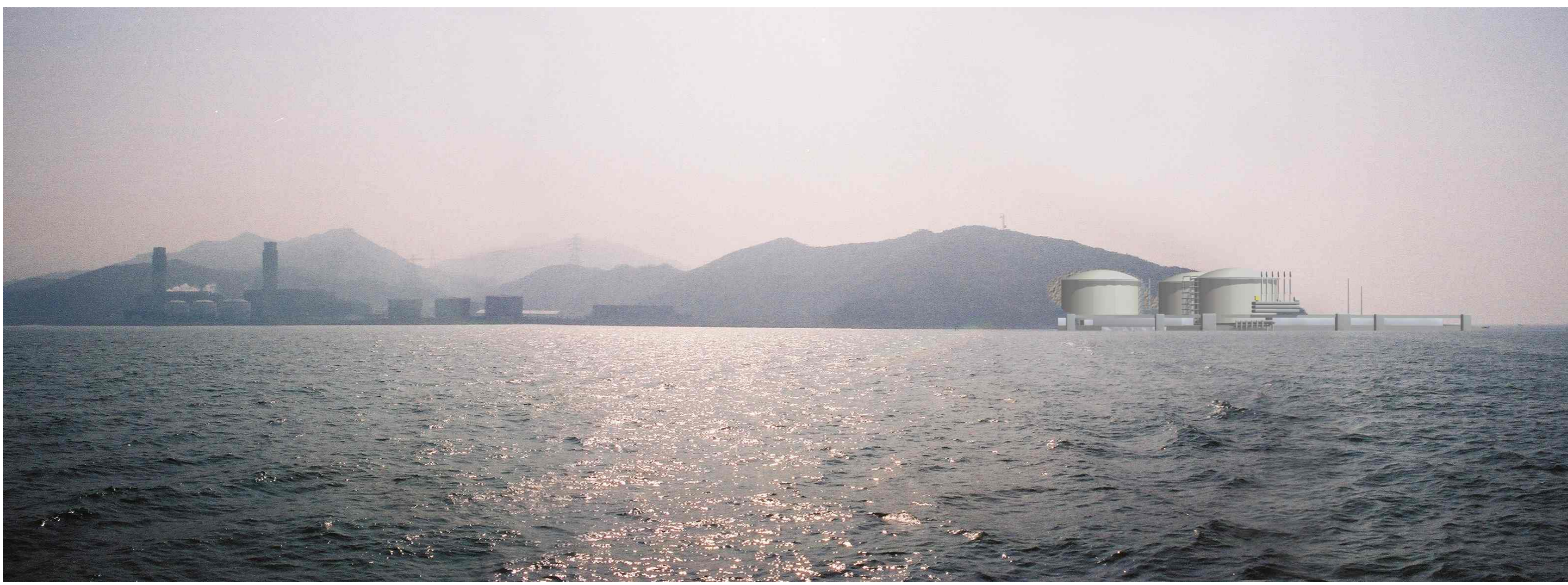
VIEW DISPLAYING THE 3D MODEL OF THE PROPOSED DEVELOPMENT DAY 1 WITH MITIGATION MEASURES
