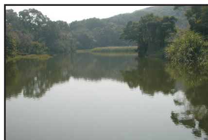
Overview of the abandoned reservoir
