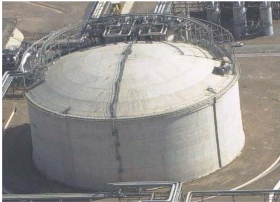
Figure 1.2 Typical LNG Storage Tank
