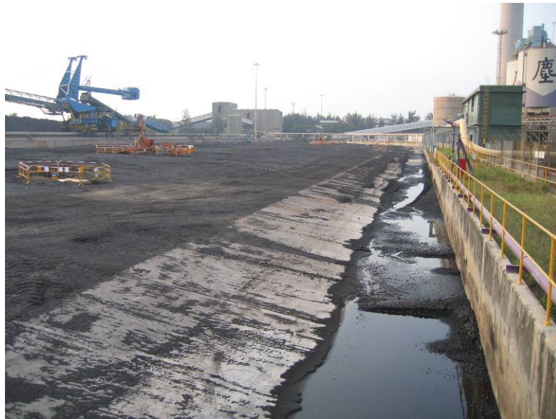
Photo P3 - North Coal Storage Yard
