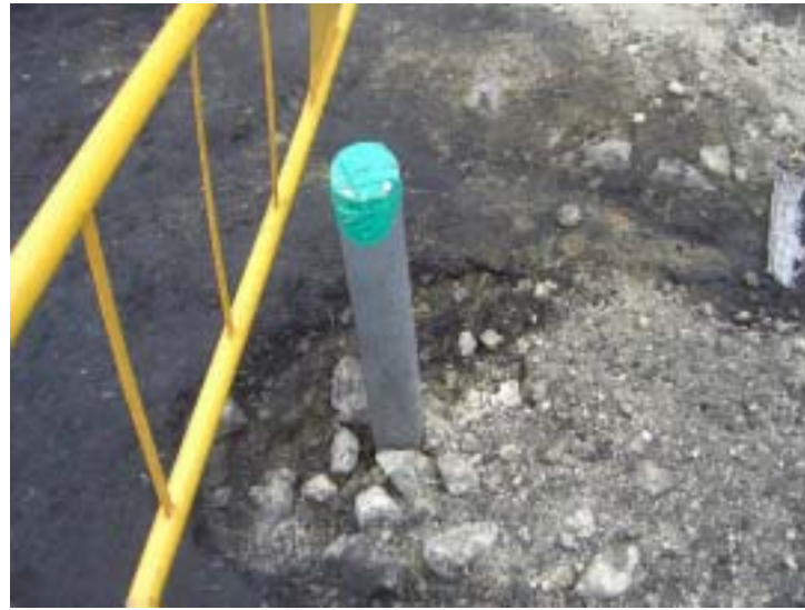
Photo 4 - Temporary groundwater sampling well installed at location DH2.
