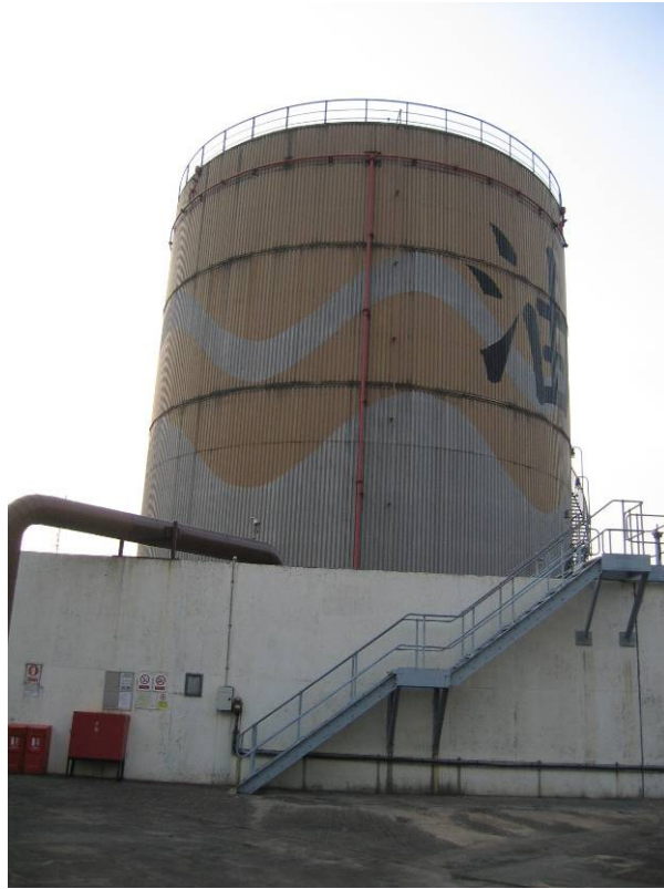
Photo P1 – Castle Peak “B” Fuel Oil Day Tank (FODT)
