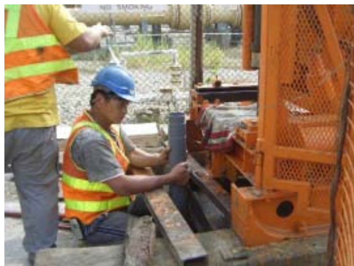
Photo 3 - Temporary groundwater sampling well installation at DH8.
