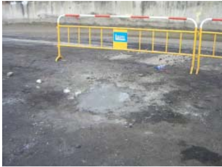
Photo 7 – Reinstated land contamination location DH5.
