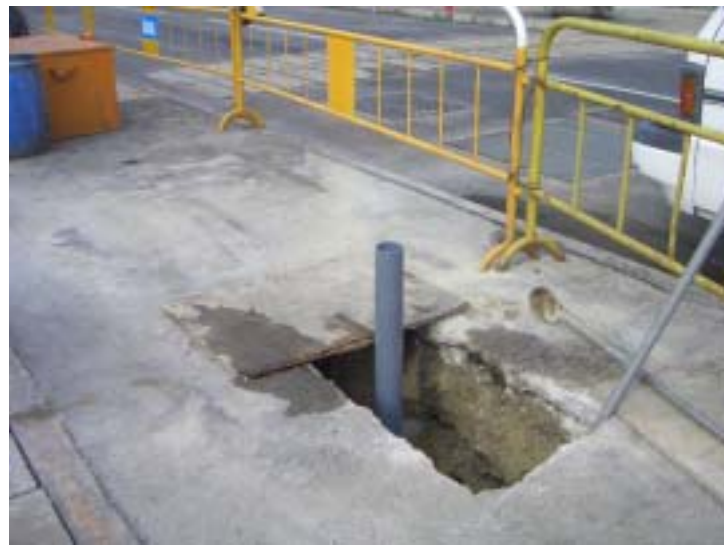
Photo 5 - Temporary groundwater sampling well installed at location DH3.
