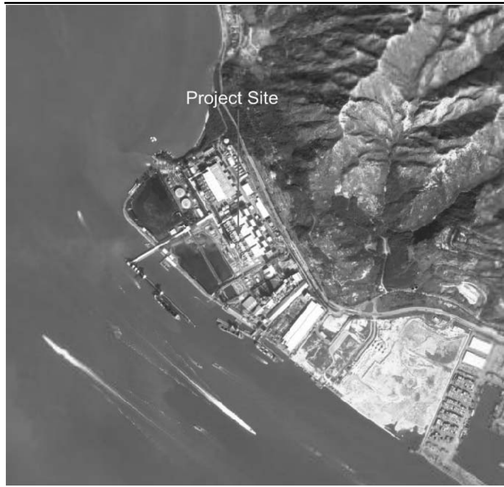
Figure 9.1 Aerial View of the Site and Its Surroundings
