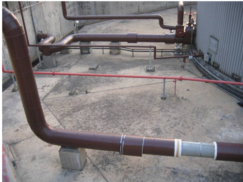
Photo P2 - Inside the FODT Bunded Area
