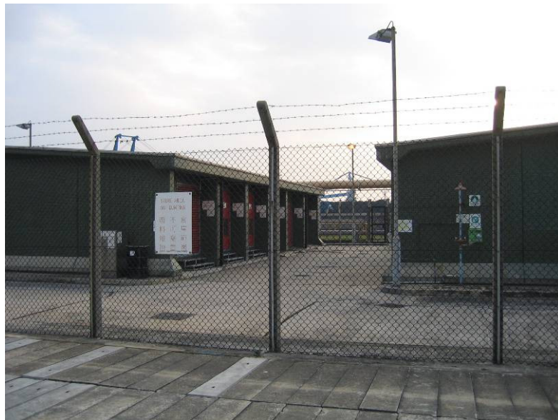
Photo P4 - Dangerous Goods Stores
