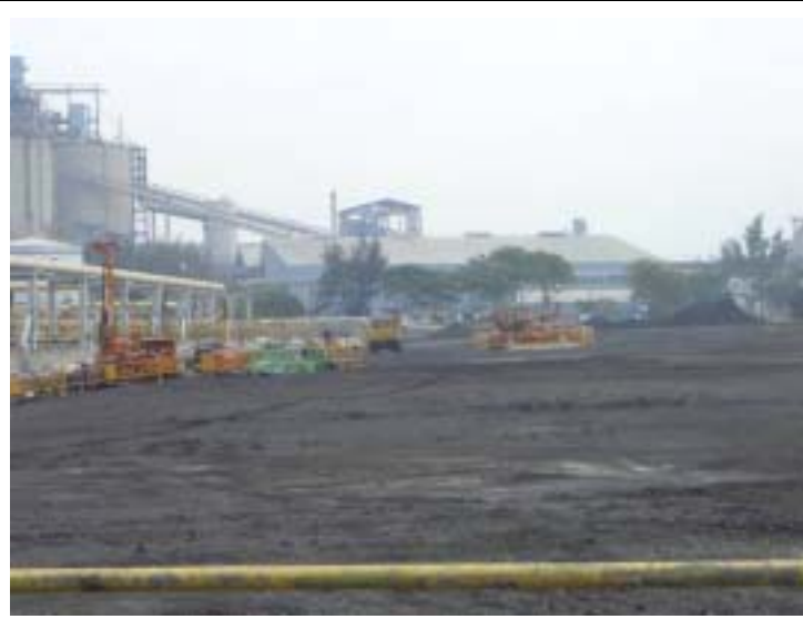
Photo 1 - Land contamination investigation at locations DH6 and DH7.
