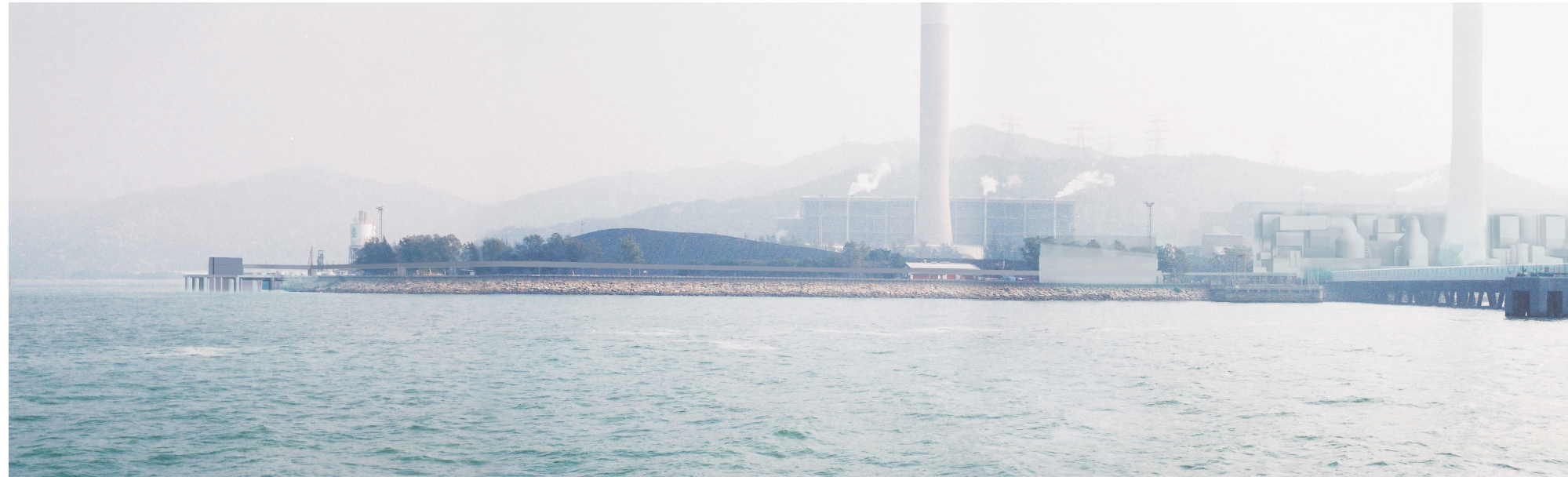
VIEW SHOWING THE EXISTING POWER STATION WITH THE PROPOSED EMISSIONS CONTROL FACILITIES.
