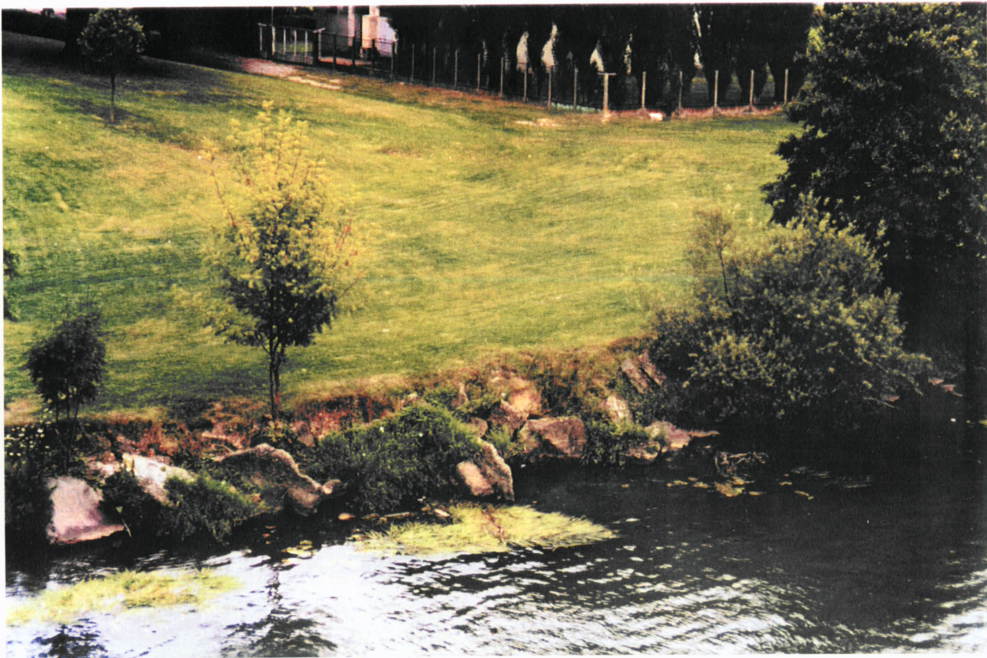
Plate 4.18 | Le Seine River near Giverny, France Rocks on Channel Margin for Protection against Erosion
