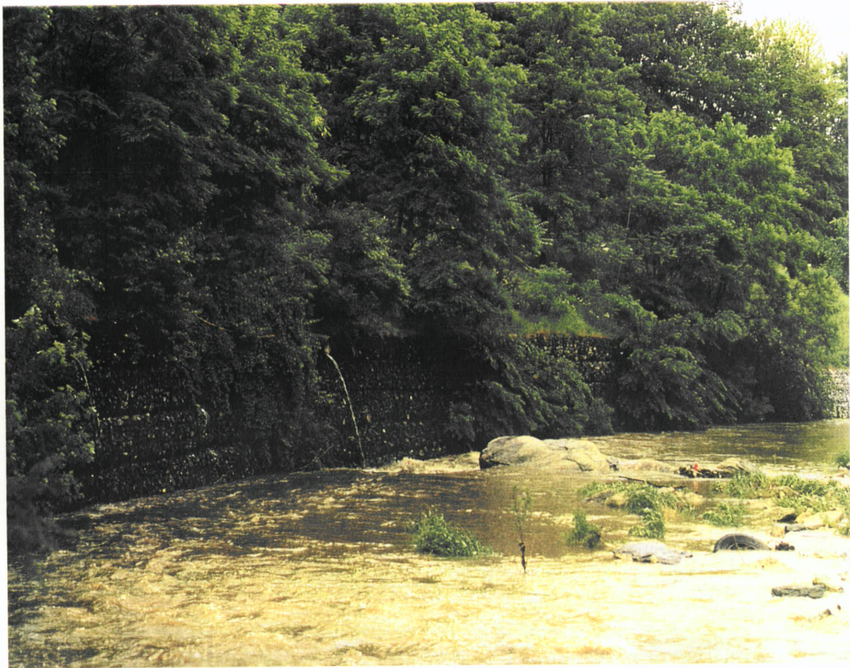
Plate 4.19 Gabion Lined River Bank in Maryland, U.S.
