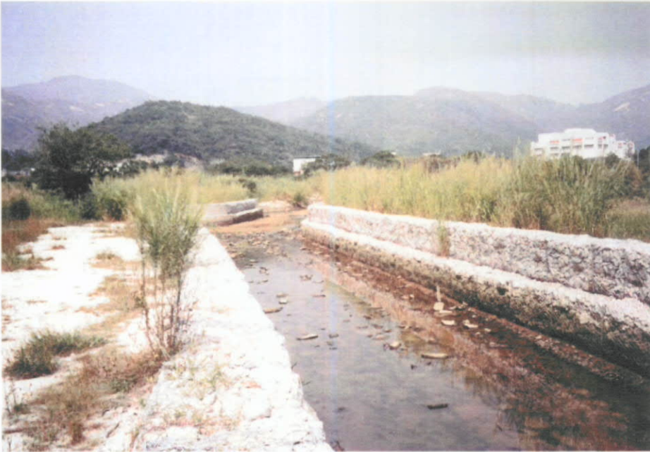
Gabion channel at Luk Tei Tong, Mui Wo, Lantau
