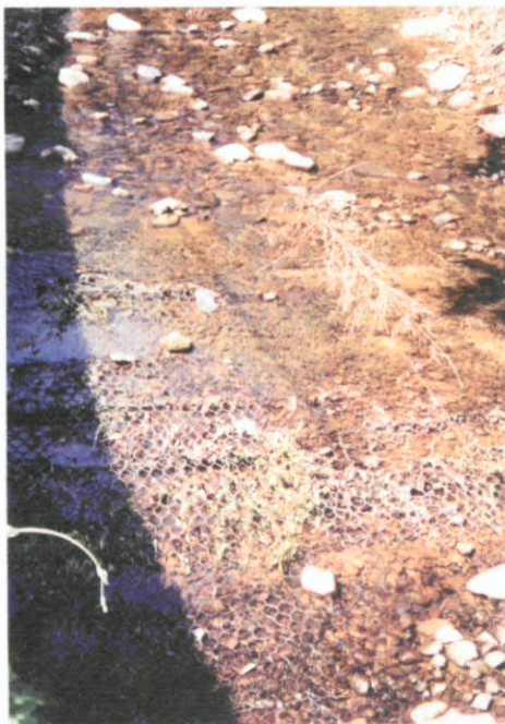
Gabion channel base
