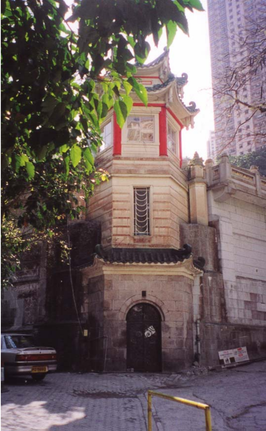
Figure 9.4 View the gate of Haw Par Mansion (from works area to the east)
