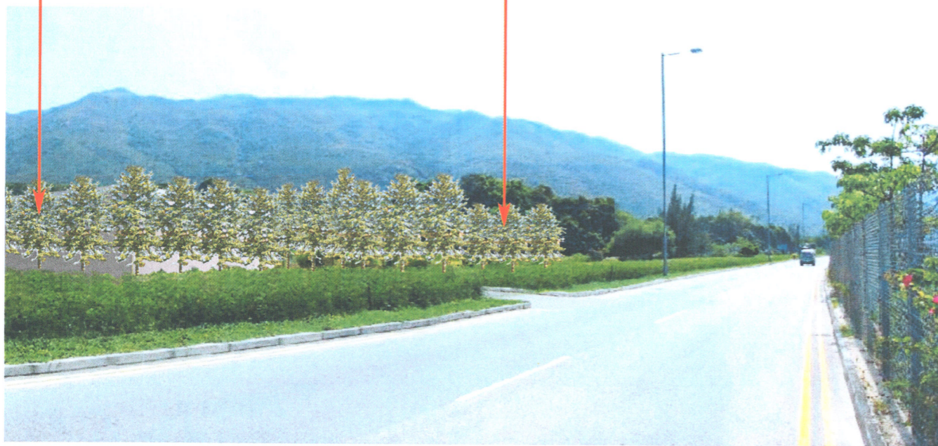
KV 1 - PROPOSED SHW RAW WATER BOOSTER PUMPING STATION YEAR 10 OPERATION WITH MITIGATION MEASURES
