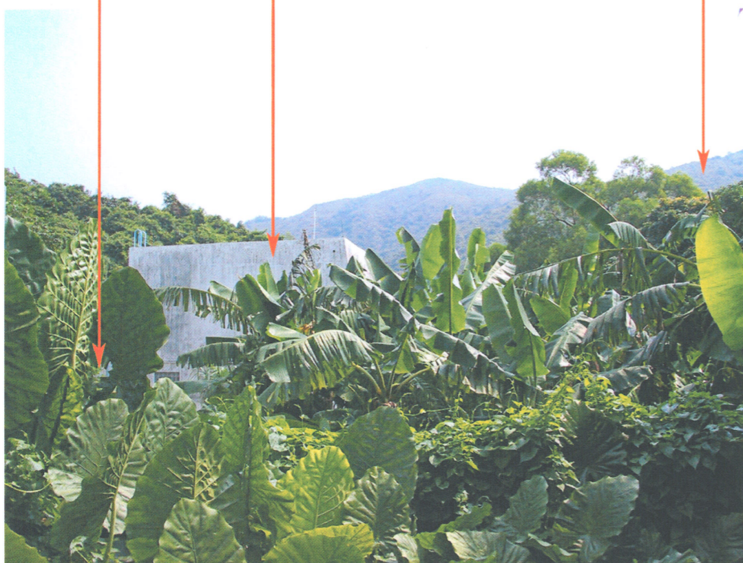
Existing View of KV 3 View from residential village house of Pui O Lo Wai Tsuen towards Existing Pui O Raw Water Pumping Station.
