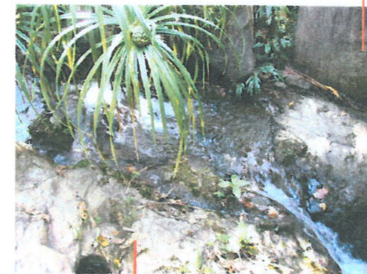
VIEW 18 Fresh water stream runs underneath South Lantau Road (LR 5)
