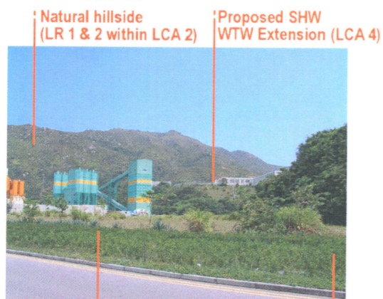
VIEW 5 Proposed SHW Raw Water Booster Pumping Station (LCA 4) Vegetated Amenity Area without trees (LR 3 within LCA 2)
