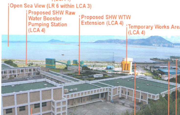
VIEW 10 SHW Water Treatment Works Area (LCA 4) Refuse Transfer Station (LCA 4)
