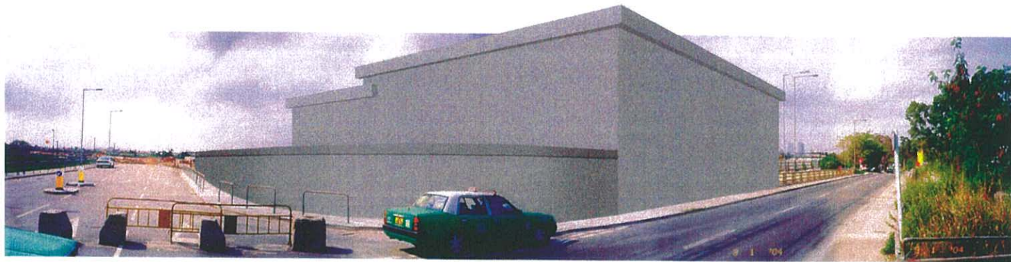
PUMPING STATION - WITHOUT MITIGATION MEASURES
