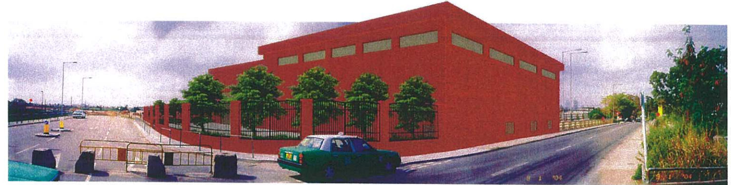
PUMPING STATION - MITIGATION MEASURES, DAY 1
