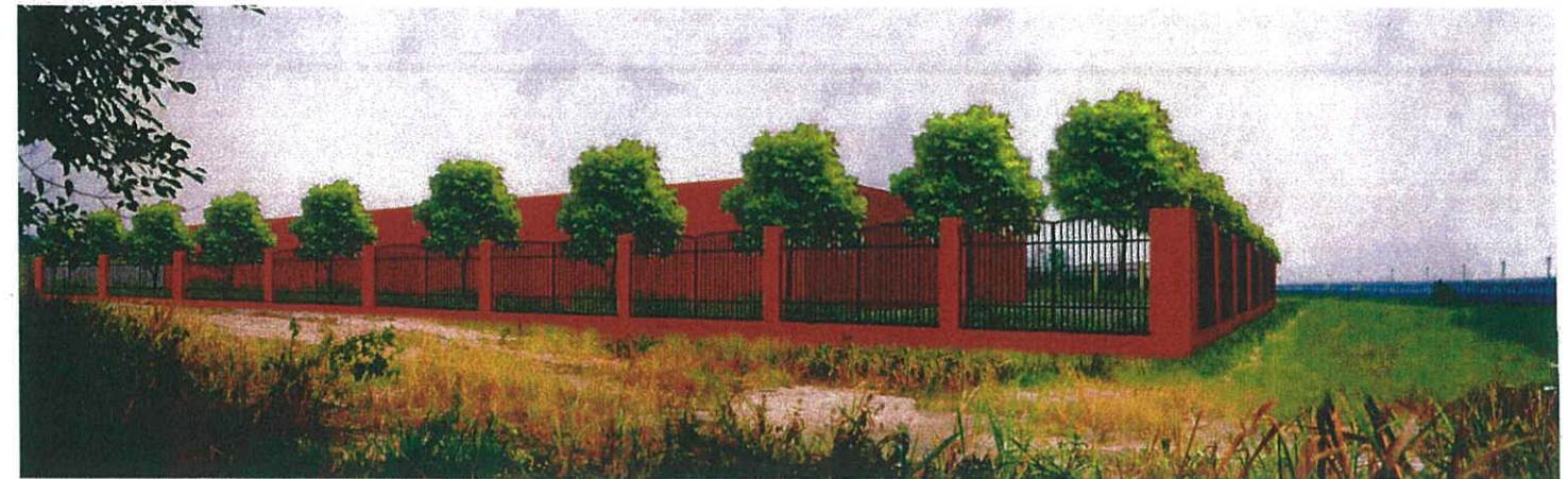
PUMPING STATION-MITIGATION MEASURES, DAY 1
