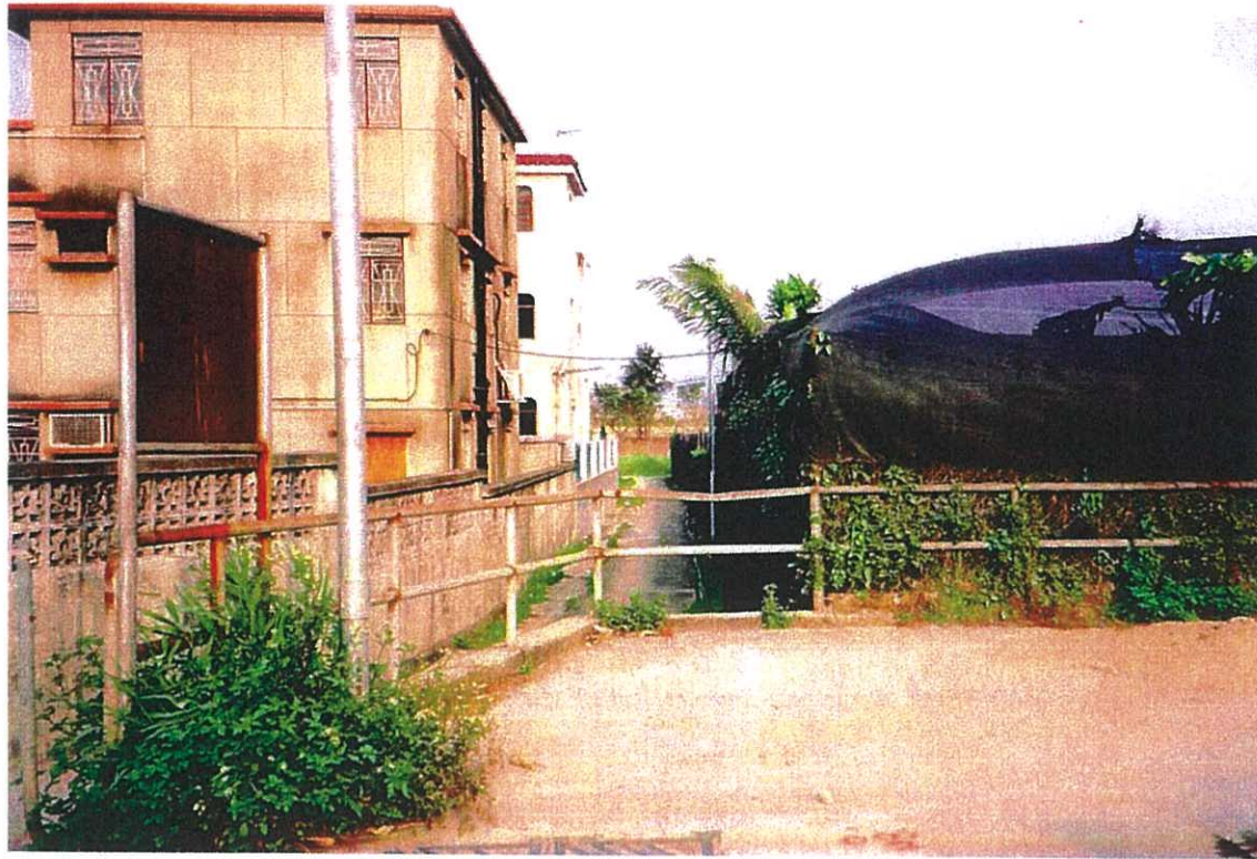
PV33: View east down route for proposed pipeline in Shan Ha Tsuen Village.
