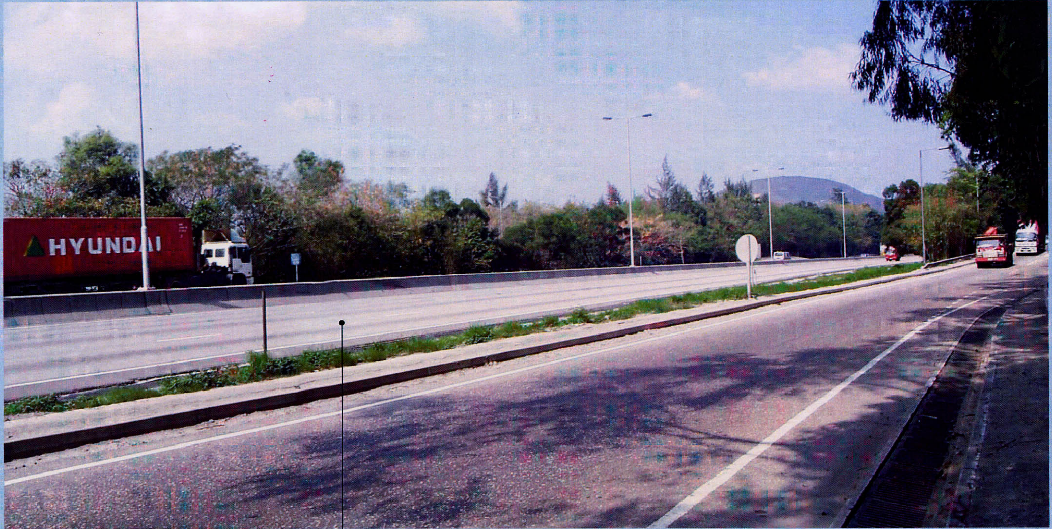
San Tin Highway
