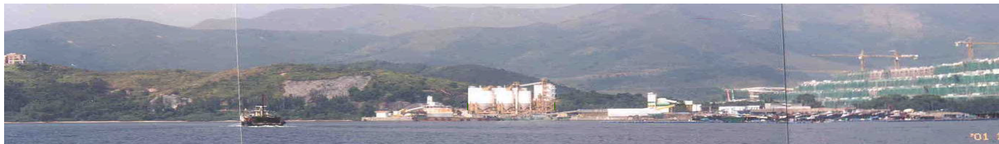
Figure 7.6c Photomontage showing view from Tolo Harbour (VSR 4) towards the site (after the project with mitigation measures option A).
