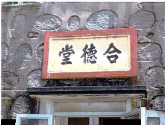
4. Horizontal Board of Left Room (1918)
