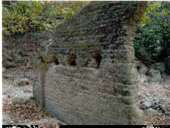
3. A Close-up View of the Remaining Wall
