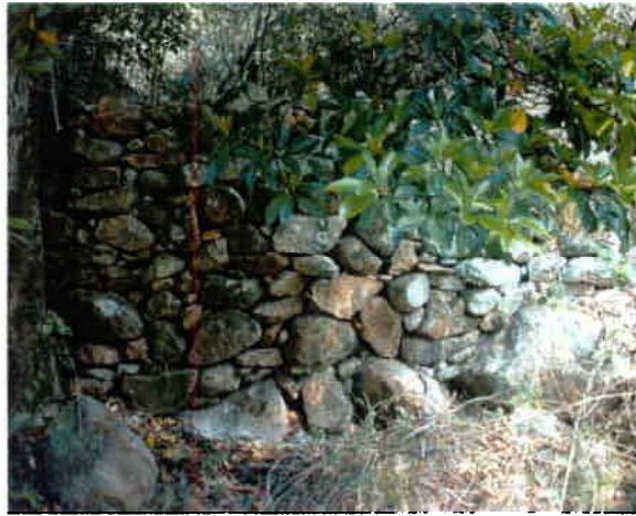
1. Stone Wall (Ruin 28)
