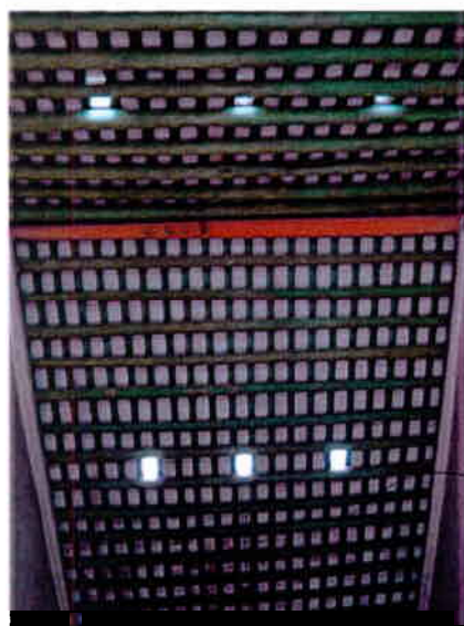
5. Frame of Rafters on Roof
