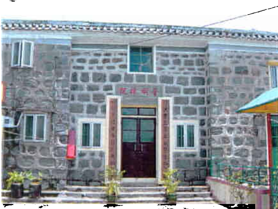
3. Front View of Middle Room (1915)
