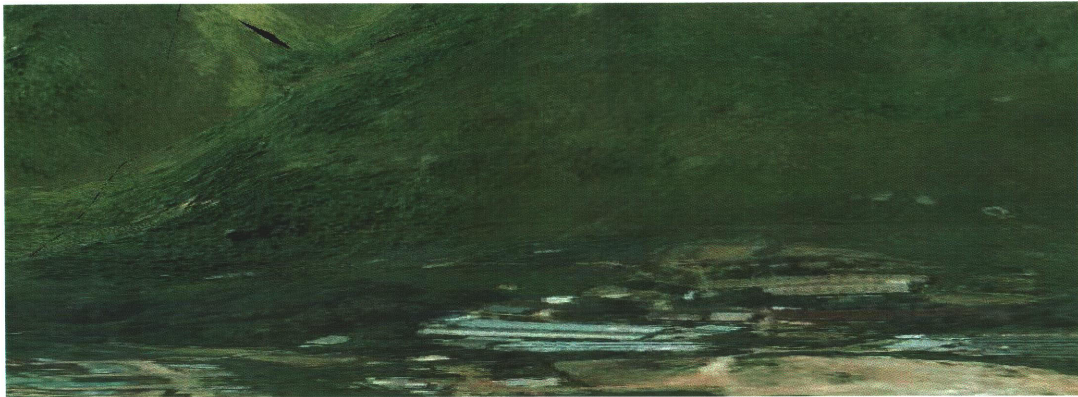
Photo View No 11 - Existing Condition
